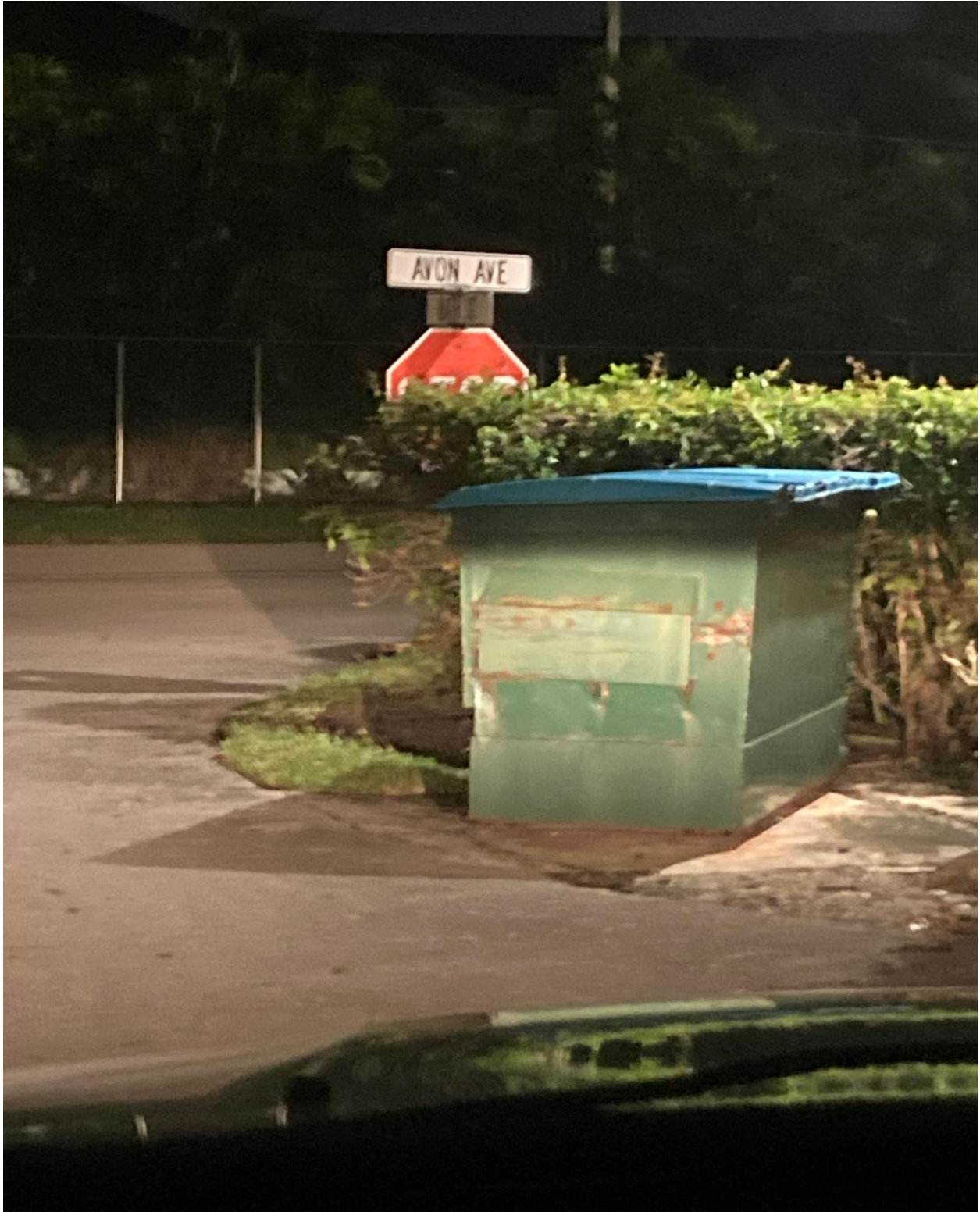
AVON AVENUE/BATH STREET- TOO SHORT STOP SIGN HIDING BEHIND A HEDGE. JOSE WILL FIX.
