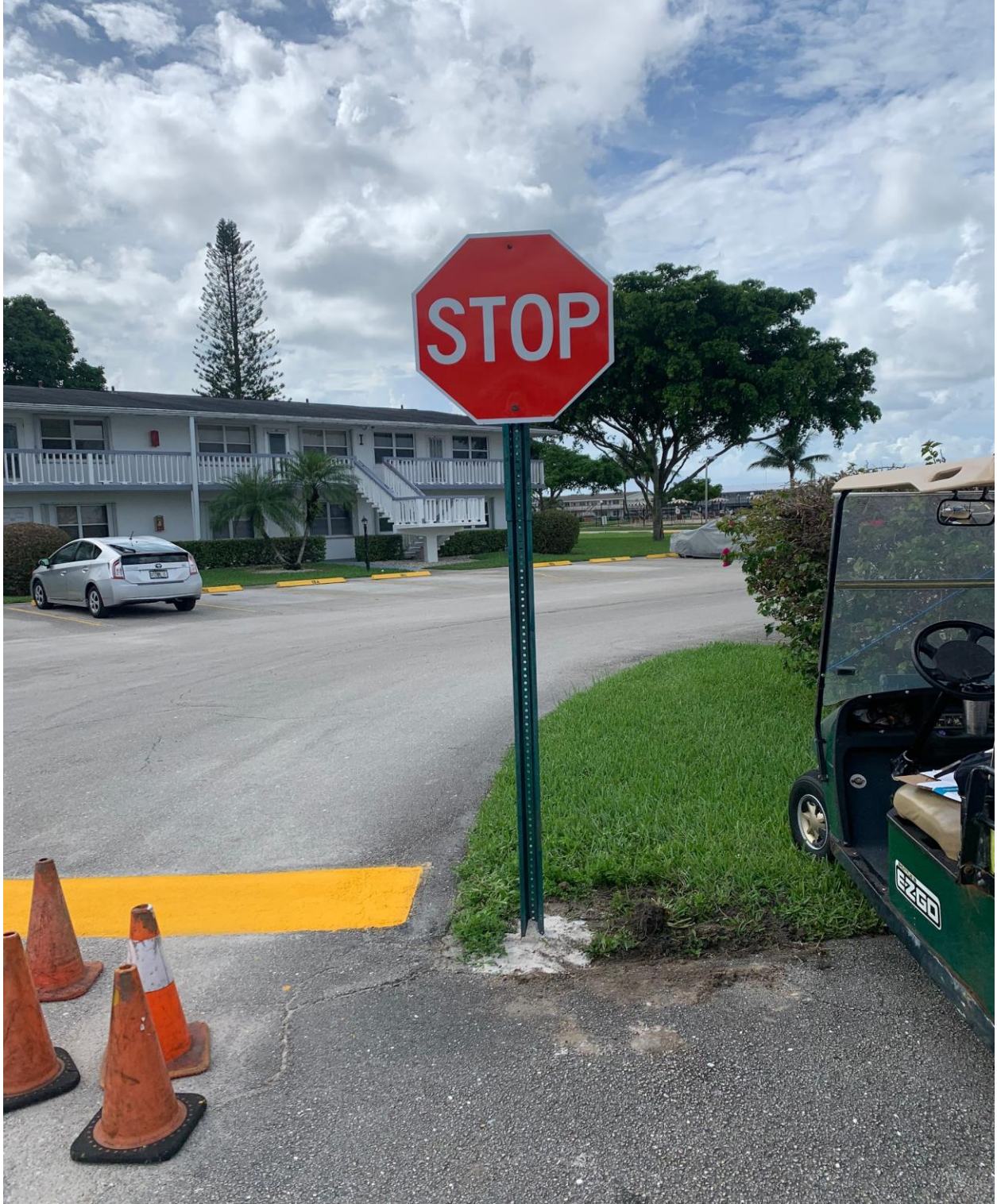
SOMERSET A- NEW STOP SIGN AND POLE. THANKS, JOSE.
