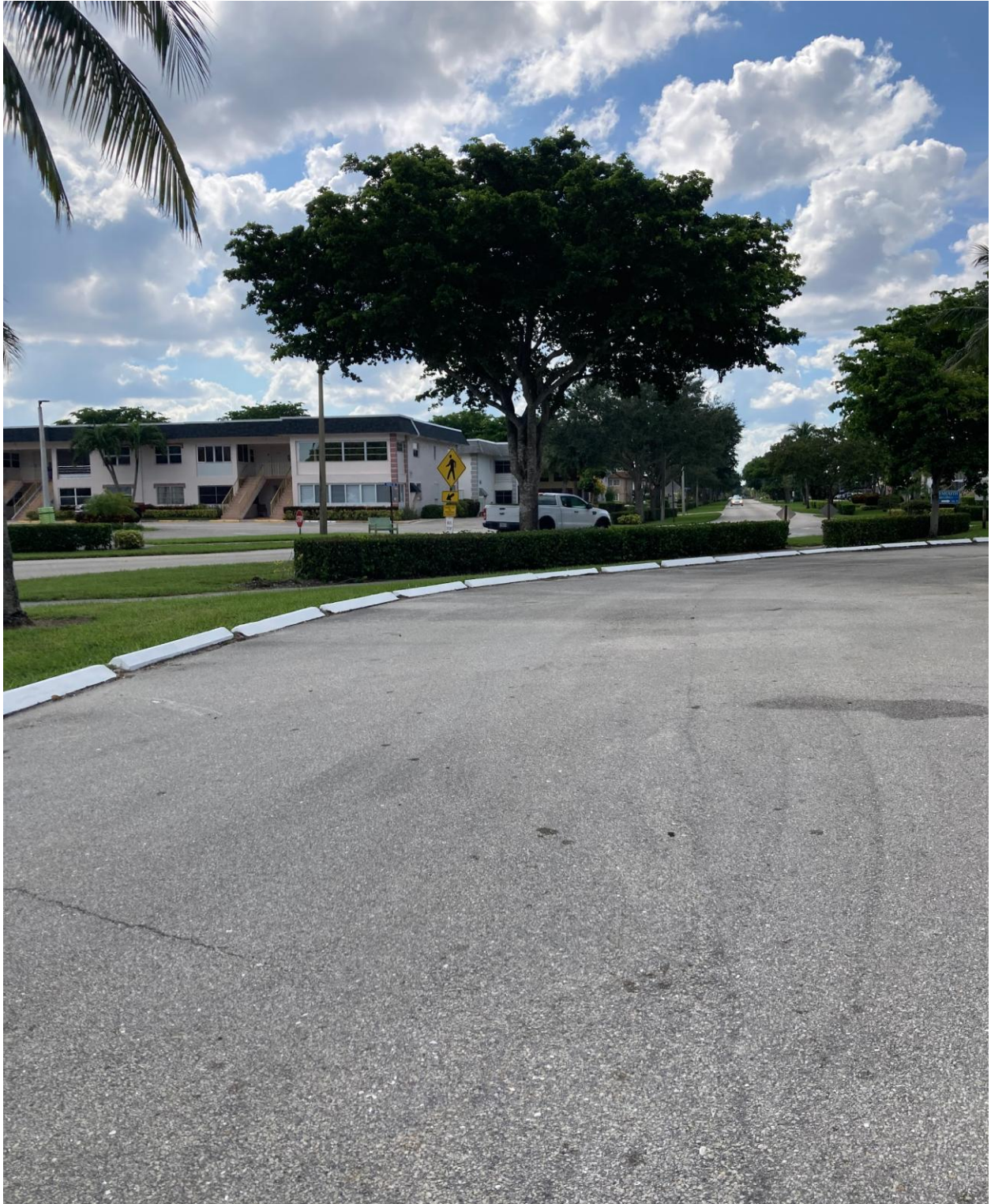
PLYMOUTH LAUNDRY- BUSTED CAR STOPS REPLACED AND ALL REPAINTED BY SEACREST SERVICES.
