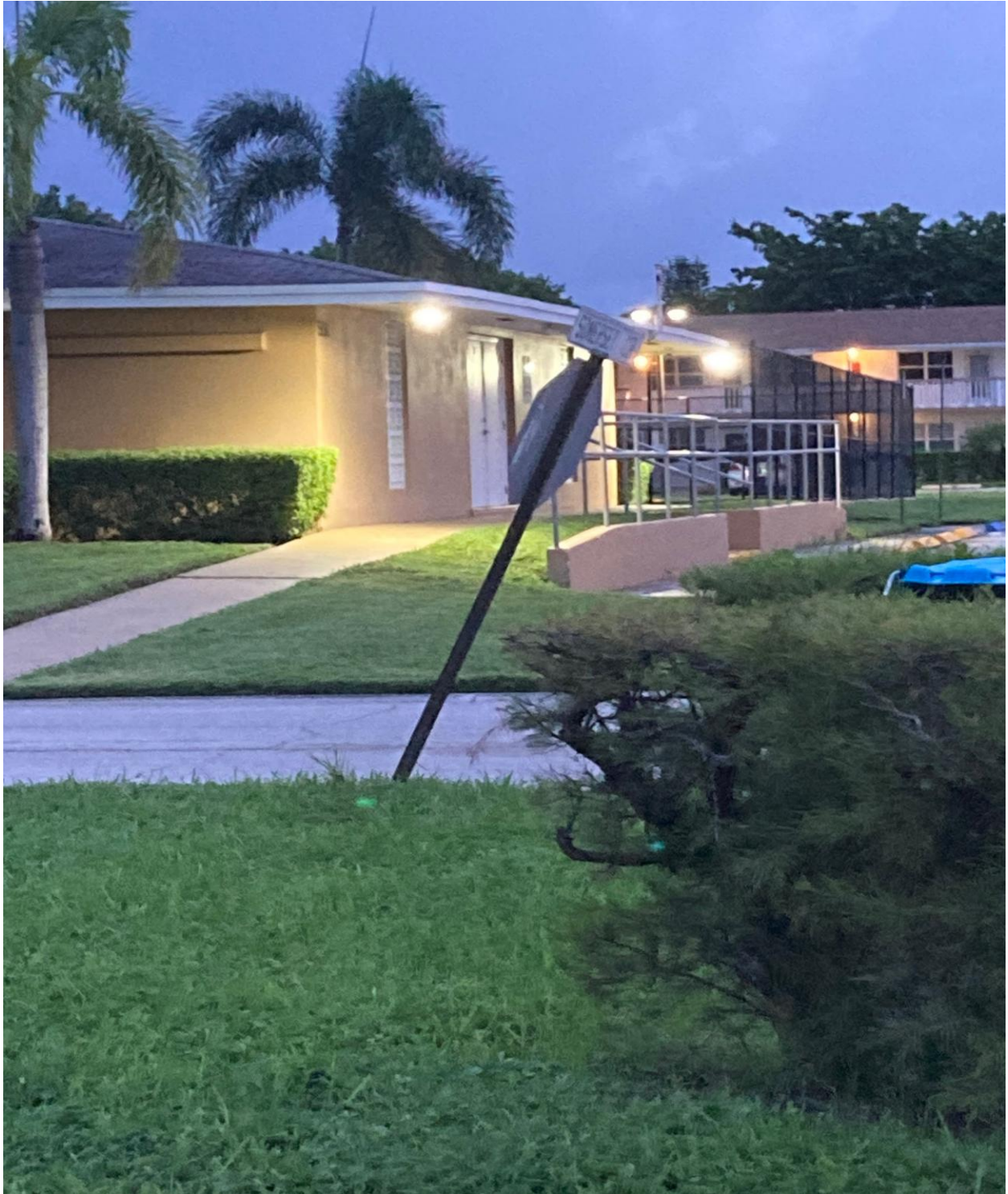
SOMERSET SECTION- THIS STOP SIGN WAS KNOCKED OVER. JOSE WILL INSTALL A NEW DOT COMPLIANT SIGN AND POLE.
