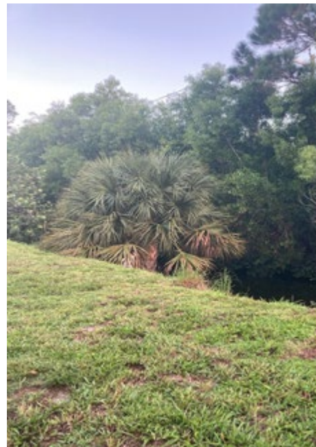
NORTH CANAL- TREES AND PALMS GROWING OUT OF THIS CANAL ARE IMPEDING MOVEMENT OF WATER AND REDUCING THE CANAL'S ABILITY TO HOLD STORM WATER. UCO DOES NOT OWN THIS CANAL, BUT OUR STORMWATER PIPES DUMP WATER INTO IT, SO WE WILL NEED TO ADDRESS THIS NUISANCE FOR SAFETY REASONS.
