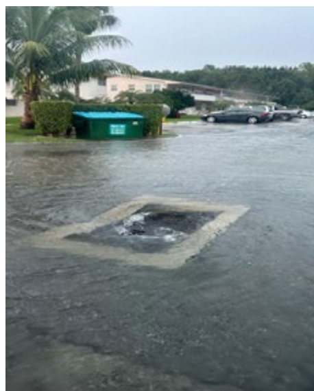
HASTINGS SECTION- HERE IS THE REASON WHY THESE CANALS NEED TO BE MAINTAINED: ALL OF OUR STORM WATER DUMPS INTO THESE CANALS. WHEN THE CANALS CANNOT ACCEPT ANY MORE WATER, THE WATER WILL BACK UP OUT OF THE CATCH BASINS AND FLOOD THE RESIDENCES. NOT GOOD. BUT UCO IS "ON IT".
