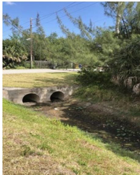
SOUTH CANAL- OVER DECADES, THIS CANAL HAS FILLED IN WITH SEDIMENT. THIS REDUCES THE CANAL'S CAPACITY TO HOLD STORM WATER. I TOOK THIS PICTURE IN 2017; THE CANAL IS ACTUALLY MORE SHALLOW NOW.
