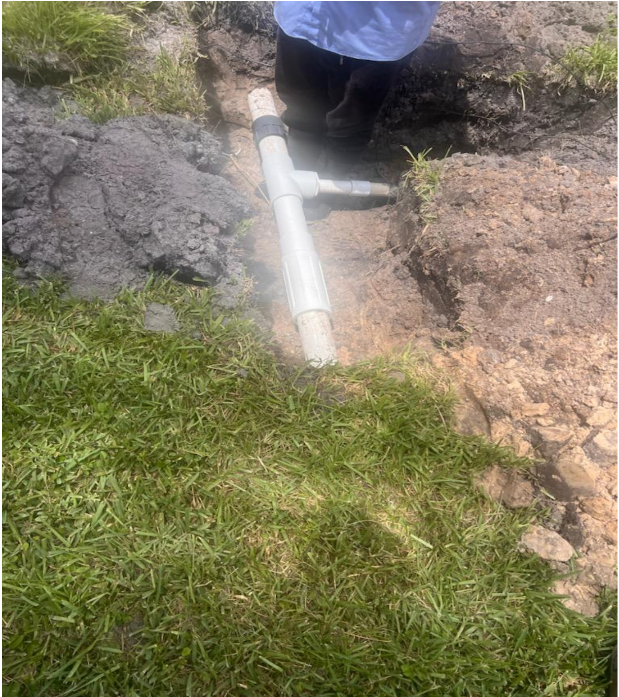
SALISBURY- THREE INCH IRRIGATION LINE REPAIRED BY SEACREST SERVICES ON 7/29.
