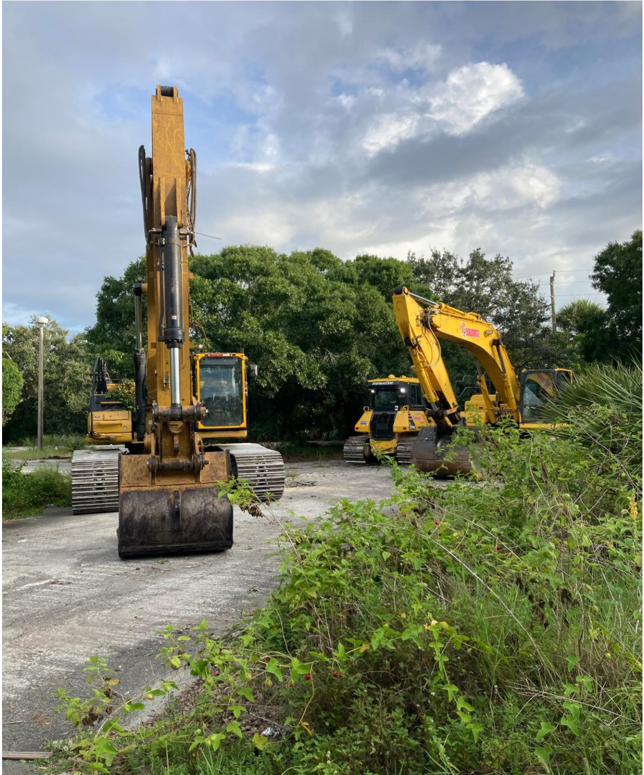
REFLECTION BAY- LAND CLEARING FOR THIS 72 ACRE PARCEL BEGAN LAST WEEK.
