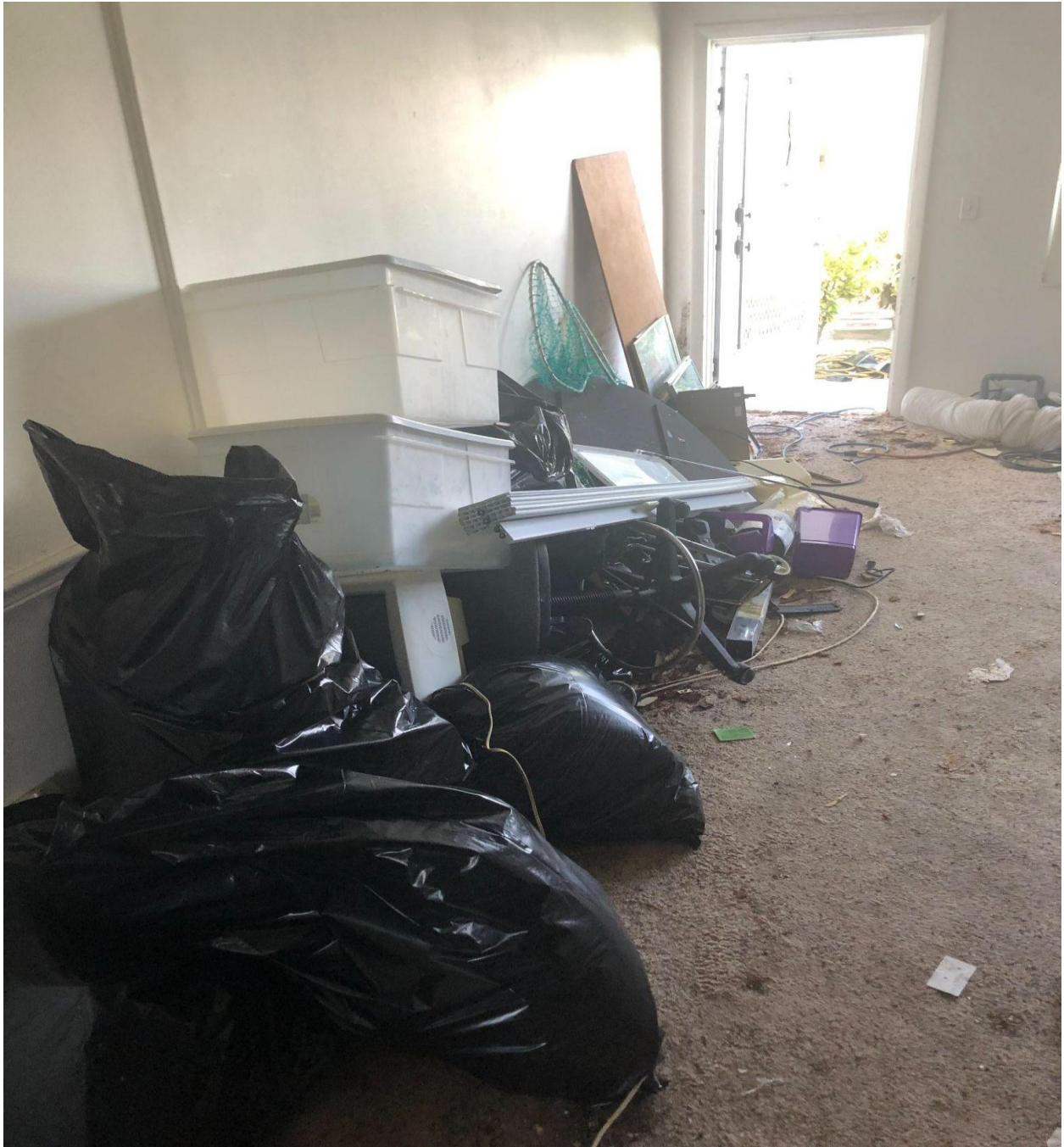
172 COVENTRY H- CONTAMINATED MATERIAL IS PILED UP AND WILL BE MOVED TO TRUCKS FOR DISPOSAL OFF- PROPERTY.
