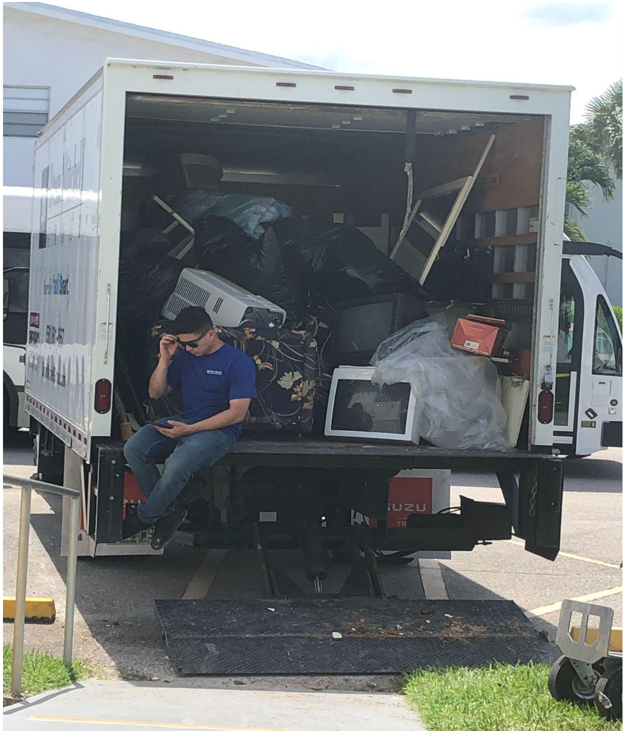
172 COVENTRY H- CONTAMINATED DEMO MATERIAL IS MOVED OFF PROPERTY BY DEAN MITCHELL.
