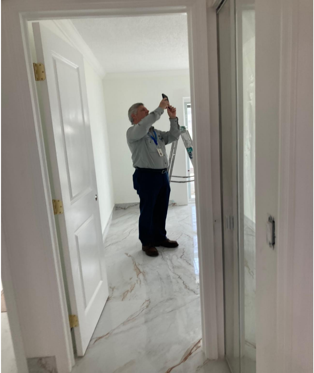
81 SOMERSET E- PZB INSPECTOR BANZHAF DOCUMENTS UNPERMITTED CONSTRUCTION WORK.
