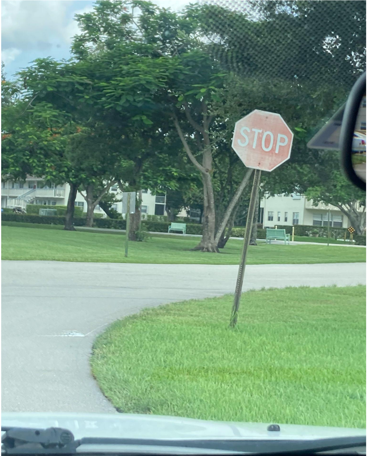
LINCOLN STREET- THIS STOP SIGN NEEDS TO BE REPLACED, AND THE SIGNPOST STRAIGHTENED OUT.
