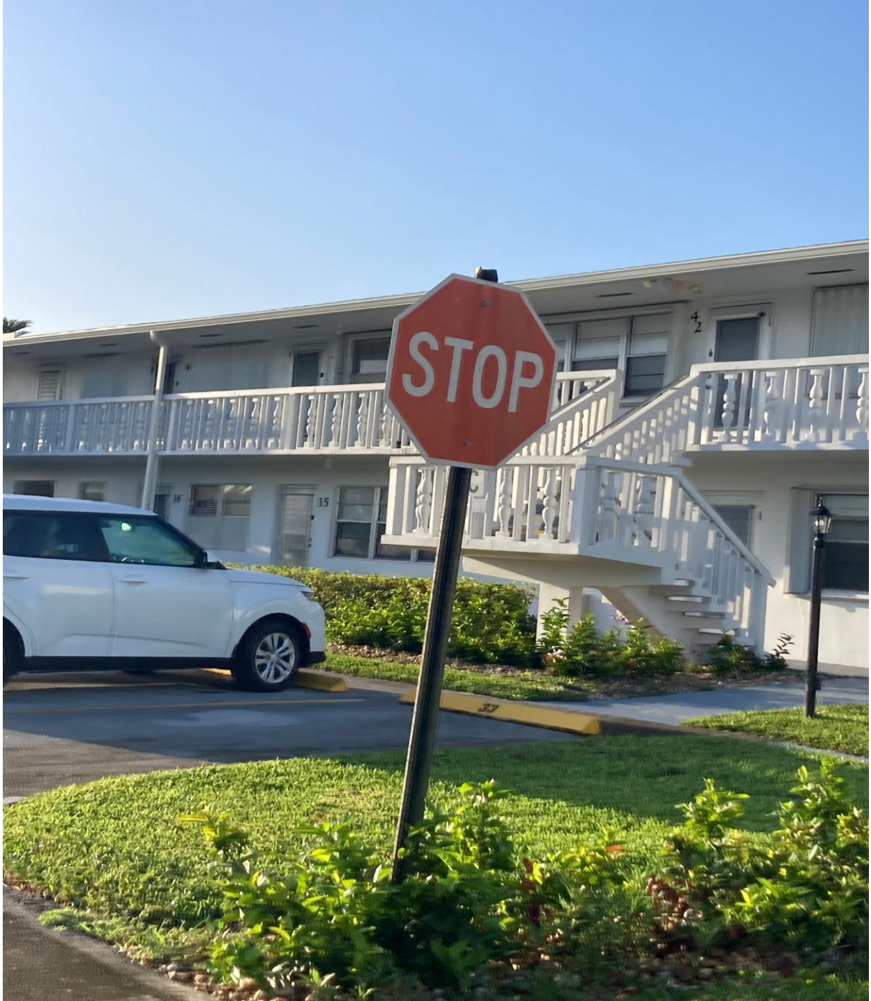
ASTOR STREET, KENT SECTION- FADED STOP SIGN, CROOKED SIGNPOST, FADED STOP BAR. JOSE WILL FIX.
