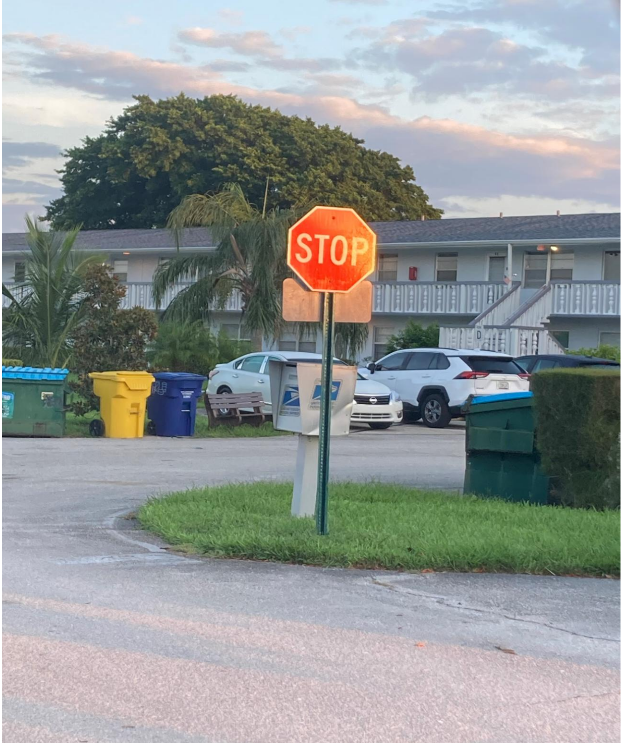
ASTOR STREET, KENT SECTION- NEW STOP SIGN INSTALLED, SIGNPOST WAS STRAIGHTENED AND PAINTED. STOP BAR WILL BE REPAINTED SOON. THANKS JOSE.
