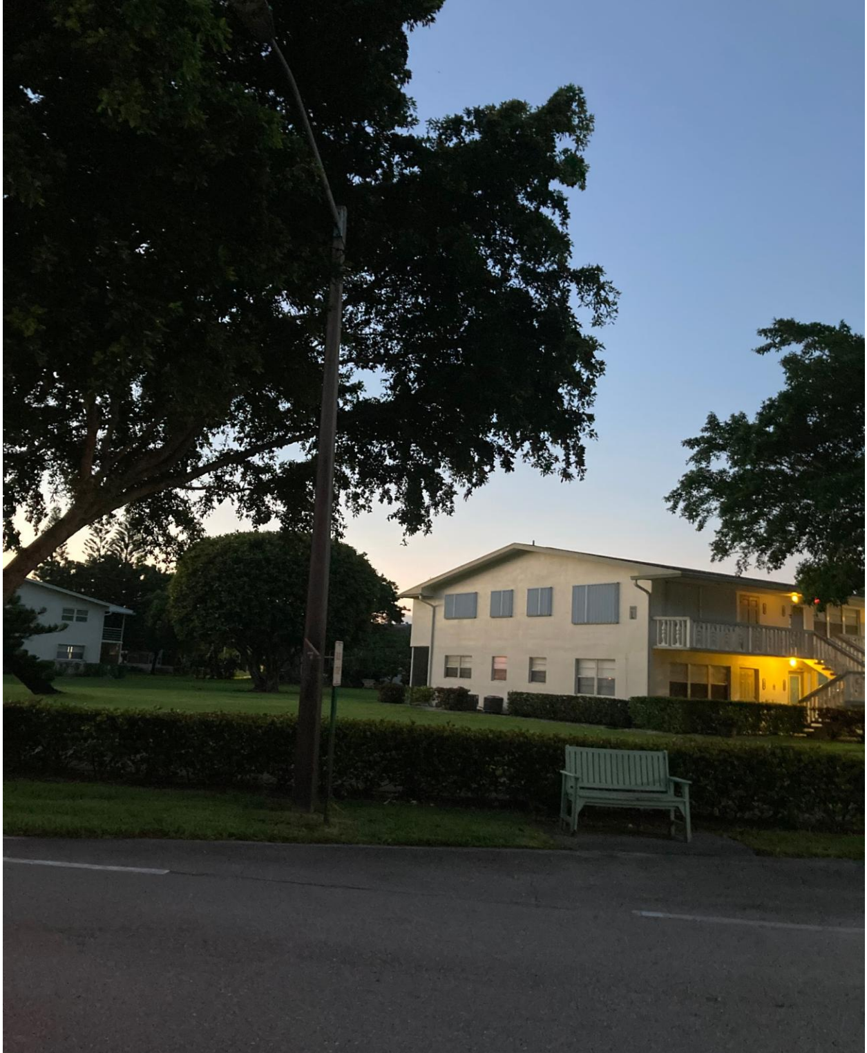
NORTH DRIVE- ANOTHER DARK STREETLIGHT. REPORTED TO FPL, WORK ORDER #42684.
