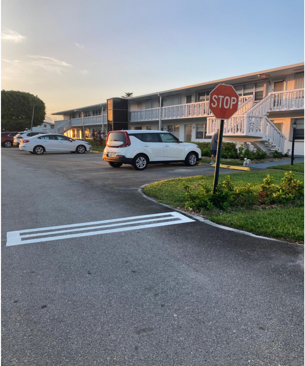
ASTOR STREET, KENT SECTION- NEW STOP SIGN INSTALLED, STOP BAR REPAINTED. THANKS JOSE.
