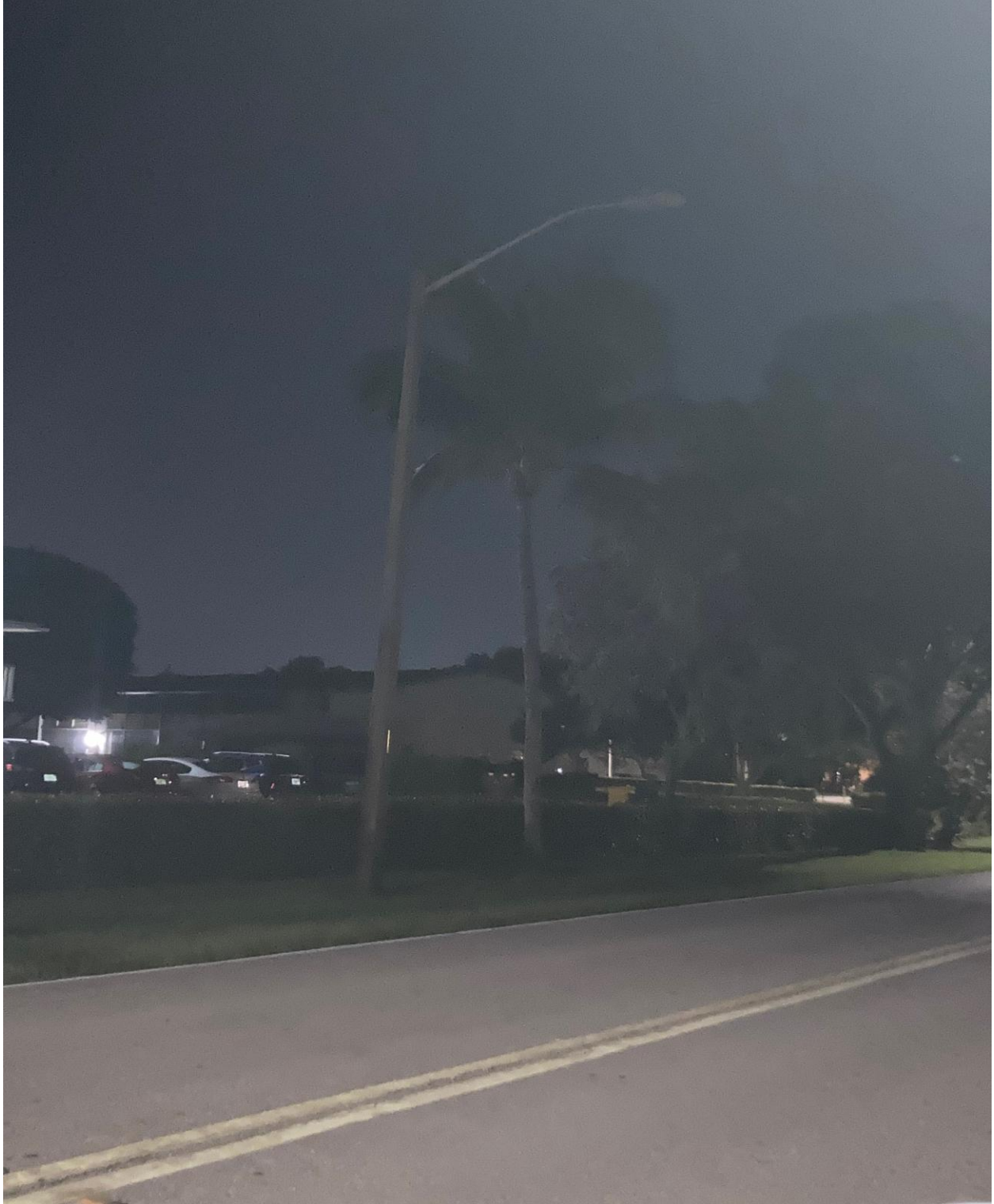
NORTH DRIVE- THIS STREETLIGHT WILL BE REPAIRED BY FPL SOON, WORK ORDER #42568.
