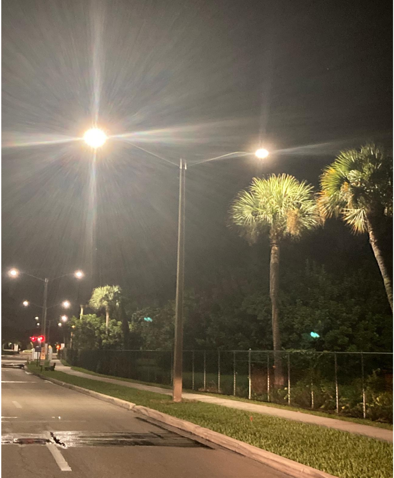
CENTURY BOULEVARD- FPL REPAIRED THIS DOUBLE STREETLIGHT ON 8/9.
