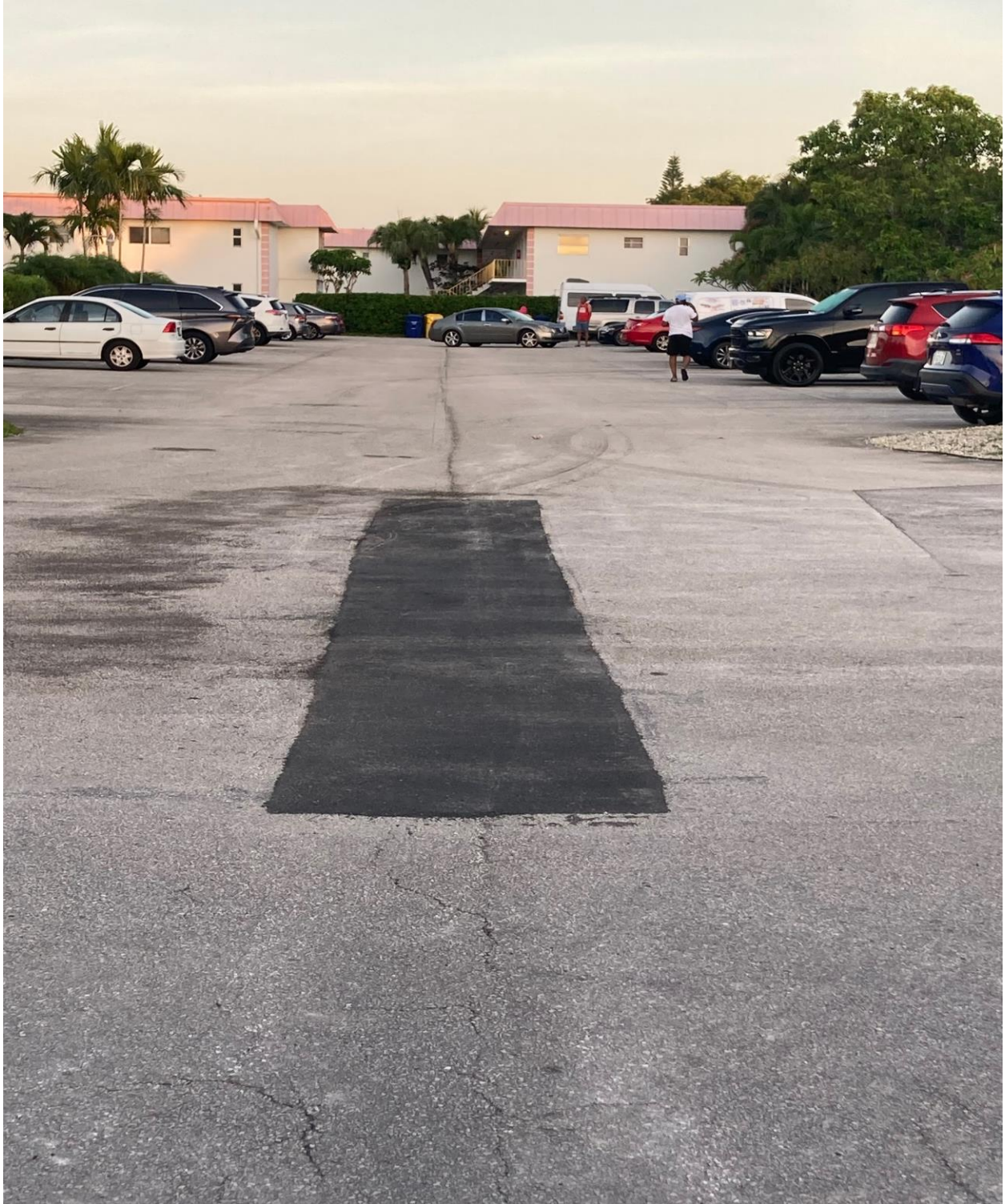
COVENTRY SECTION- ROAD REPAIR COMPLETE.
