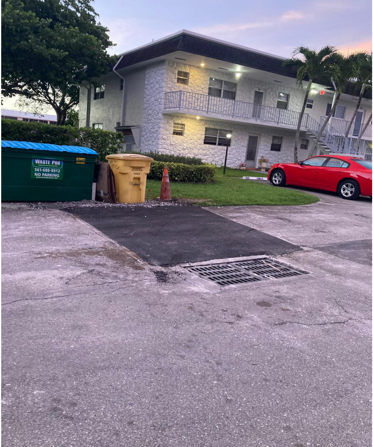
OXFORD SECTION- ROAD REPAIR COMPLETE.
