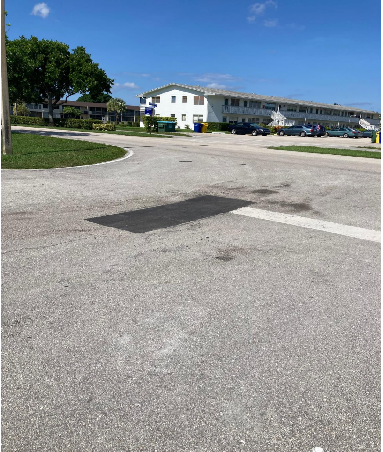
BERKSHIRE SECTION- ROAD REPAIR COMPLETE.
