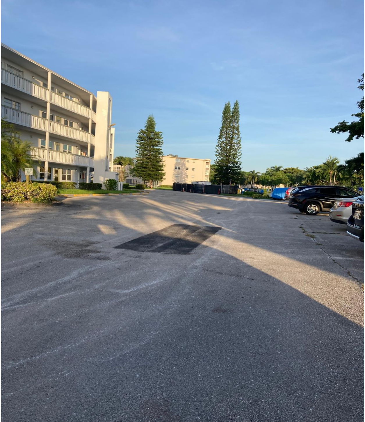
WELLINGTON H- ROAD REPAIR COMPLETE.
