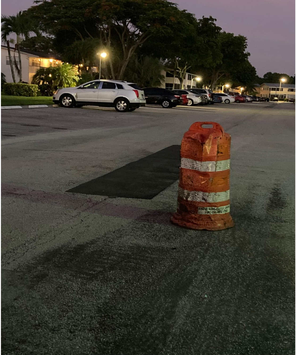
WINDSOR SECTION- ROAD REPAIR COMPLETE.
