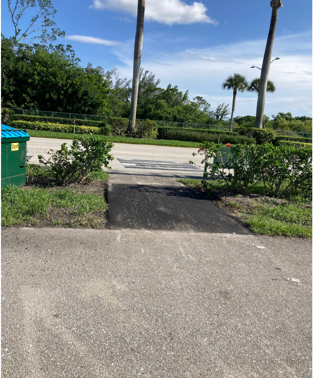
CENTURY BOULEVARD/SALISBURY A- WALKWAY REPAIR COMPLETE.
