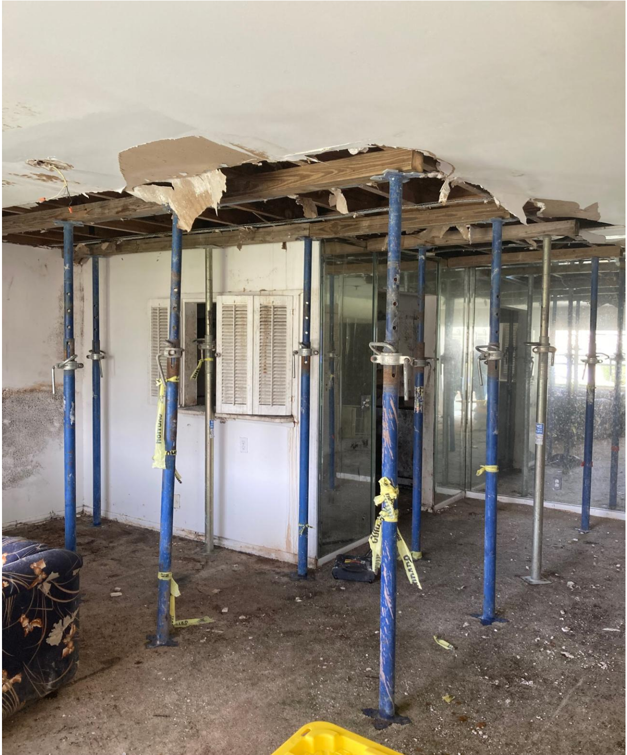
170 COVENTRY H- CR1 INSTALLED POST SHORING, WHICH WILL STABILIZE THE BUILDING.
