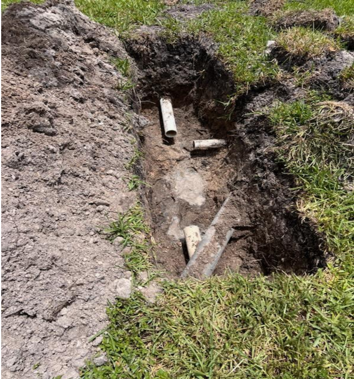
SUSSEX I- UNDERGROUND IRRIGATION SUPPLY PIPE REPAIRED BY SEACREST SERVICES.
