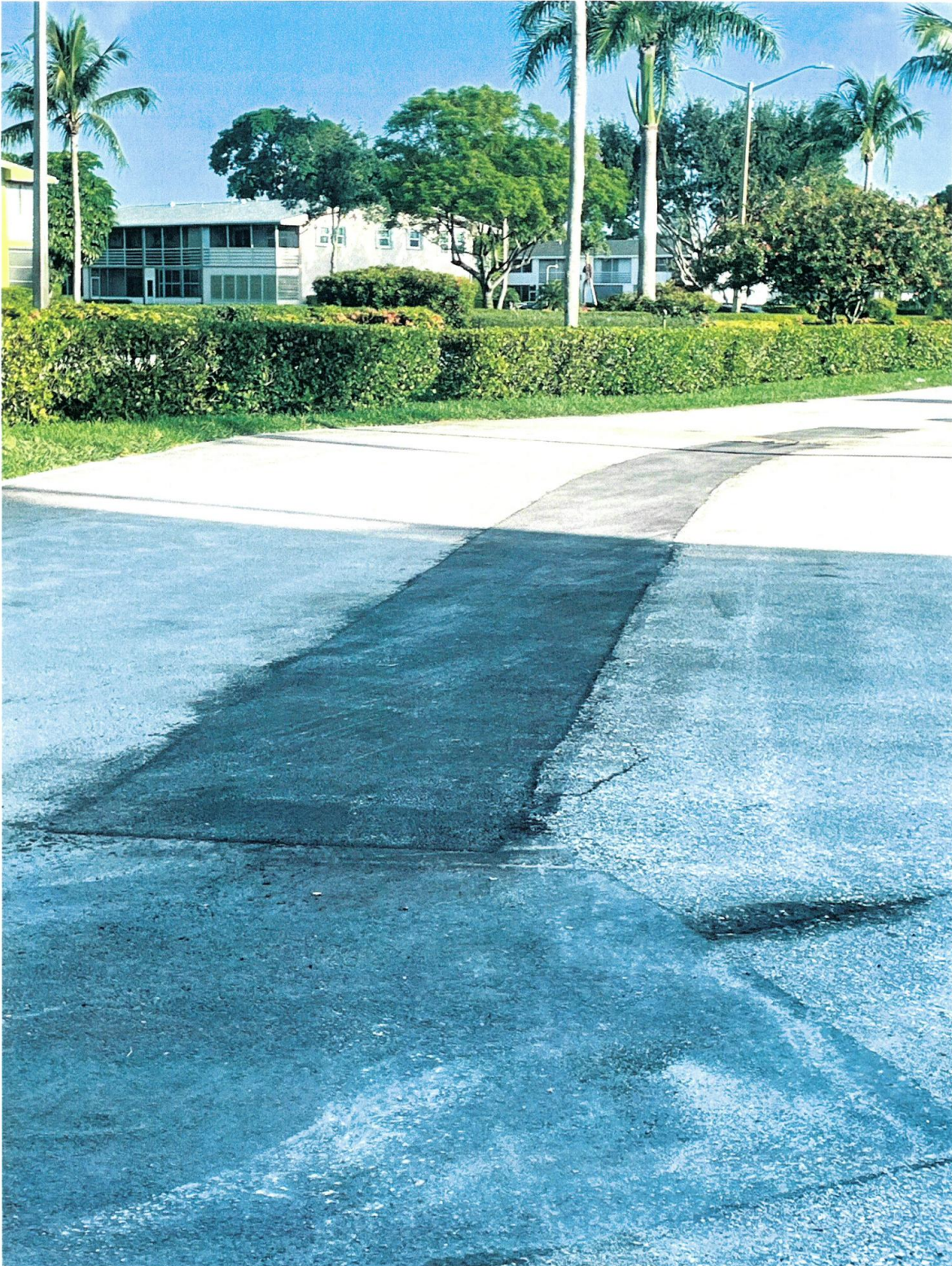
WELLINGTON SECTION- ROAD REPAIR COMPLETE.
