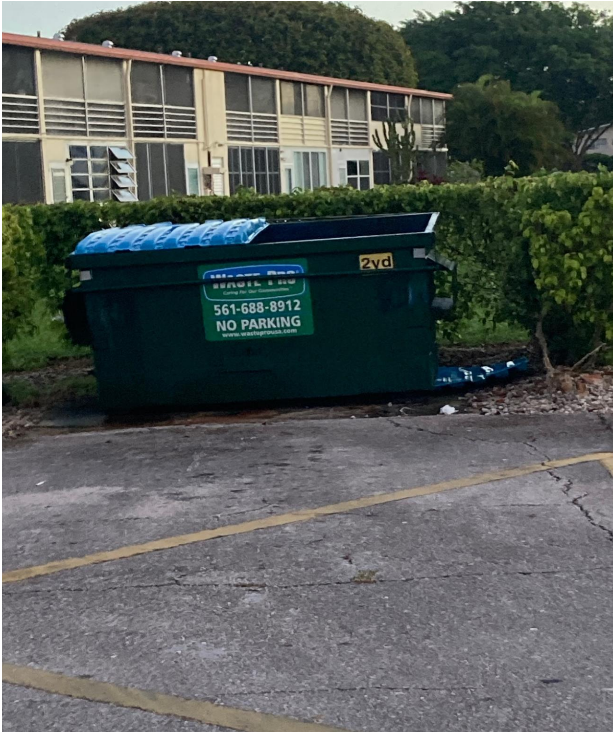
WINDSOR N- DUMPSTER WITH BUSTED LID. REQUEST FOR REPLACEMENT WAS SENT TO WASTE PRO.
