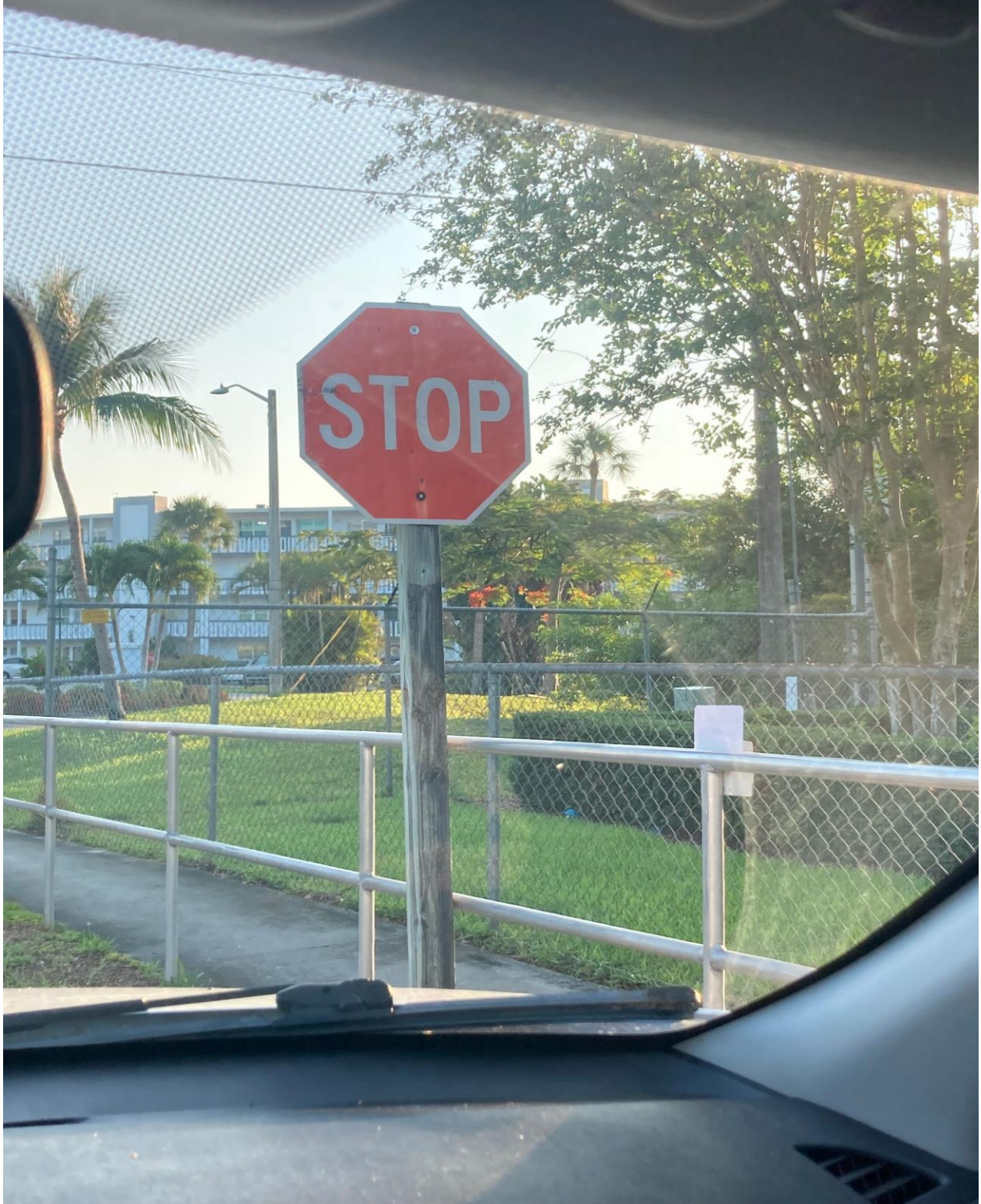
OKEECHOBEE BOULEVARD ENTRANCE- STOP SIGNS AT BOTH ENTRANCES WERE FADED, AND REQUIRED REPLACEMENT.
