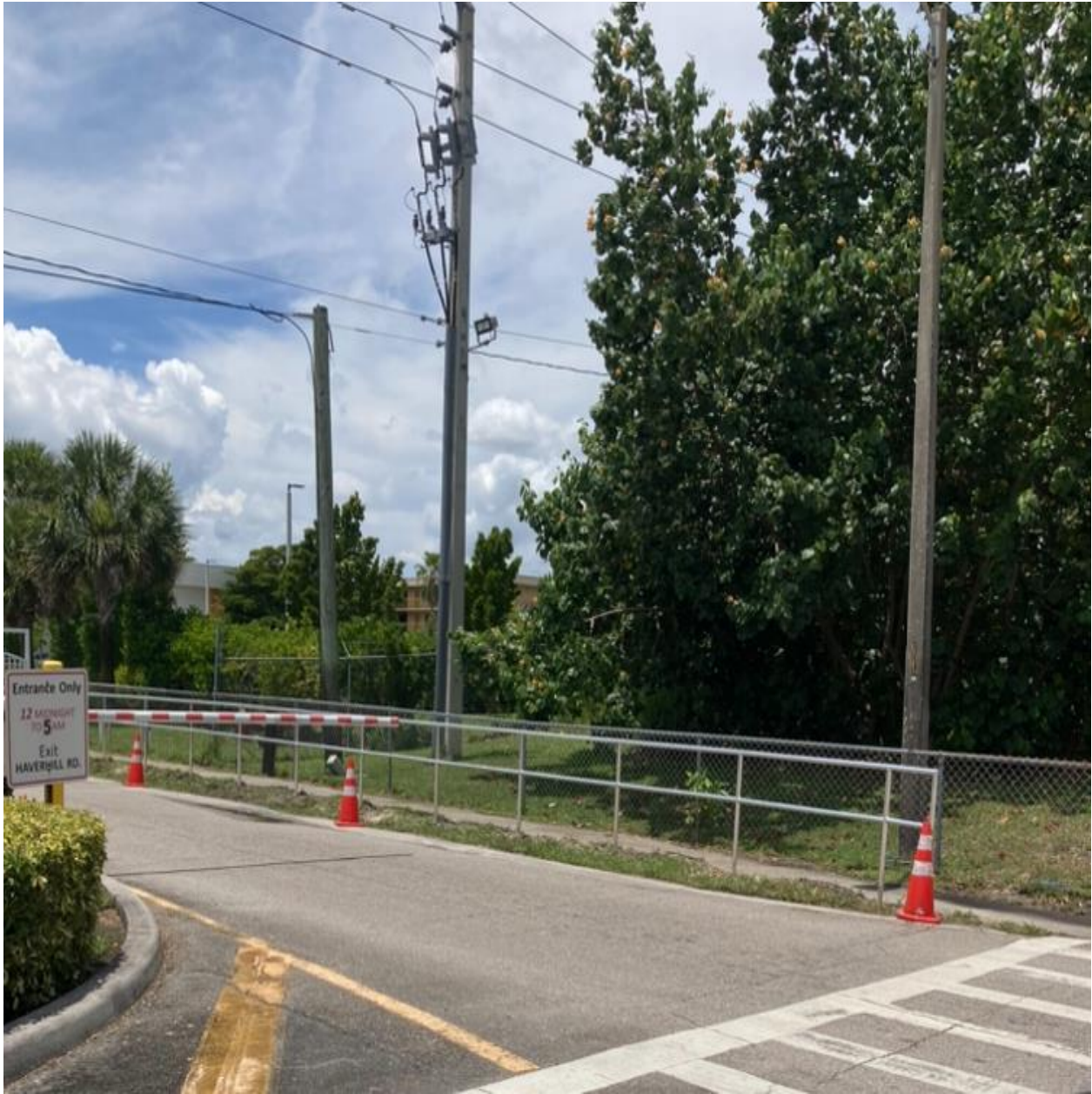
WEST DRIVE- RAILING INSTALLATION COMPLETE
