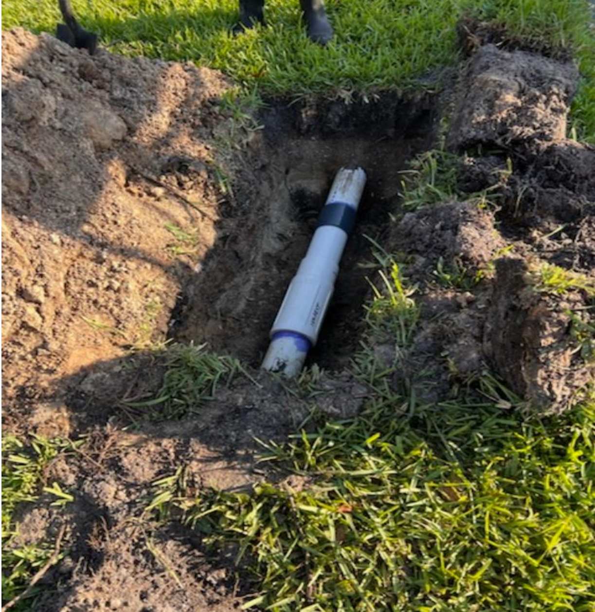
CAMBRIDGE G- FOUR INCH IRRIGATION PIPE REPAIRED BY SEACREST SERVICES ON 6/7.
