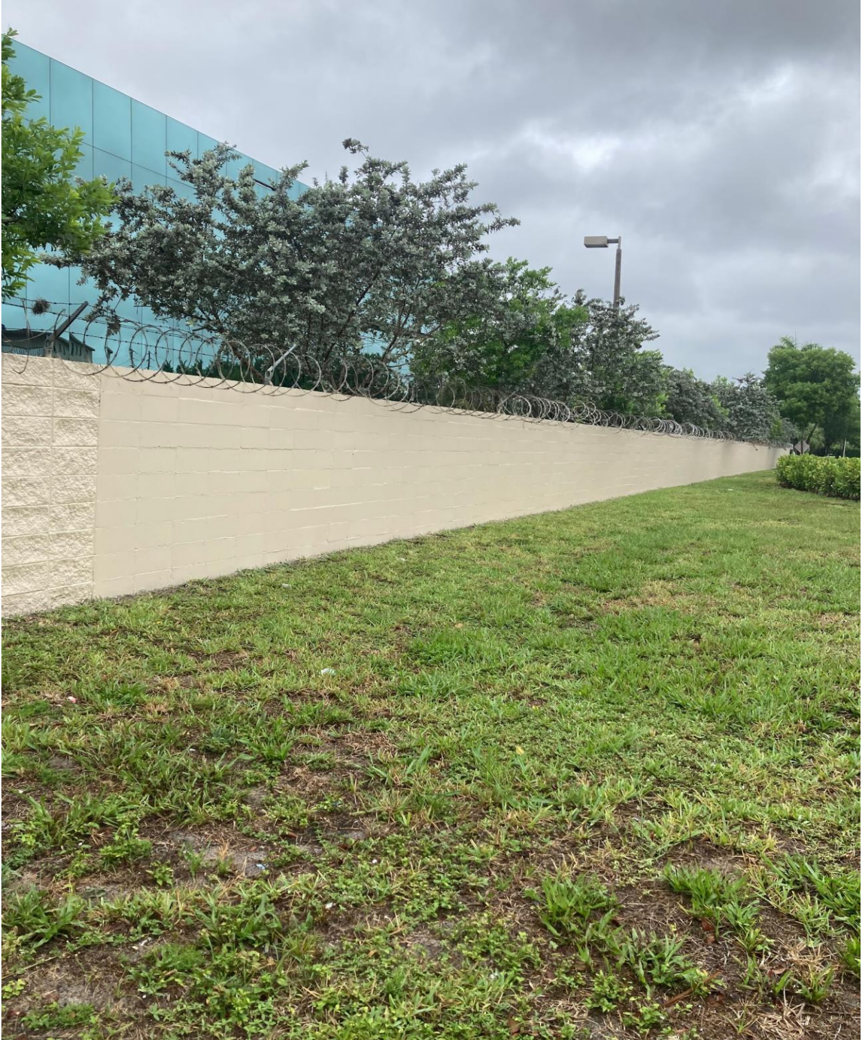
FAIRWAY STREET, SOUTHAMPTON SECTION- THIS WALL WAS PRESSURE CLEANED AND PAINTED BY PERGOLIZZI PAINTING.
