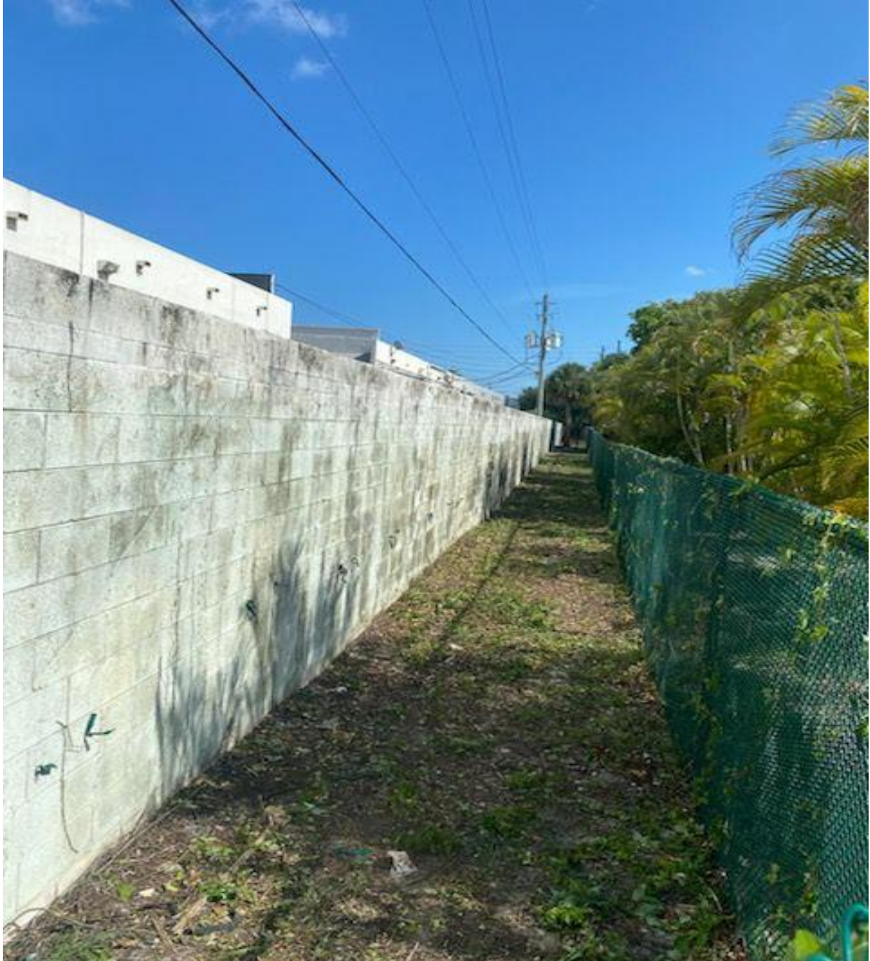
SOUTHAMPTON SECTION- PREP WORK COMPLETE, READY FOR PRESSURE CLEANING AND PAINTING.
