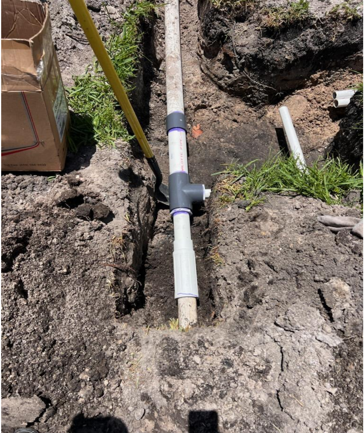
OXFORD 600- FOUR INCH IRRIGATION SUPPLY PIPE REPAIRED BY SEACREST SERVICES.
