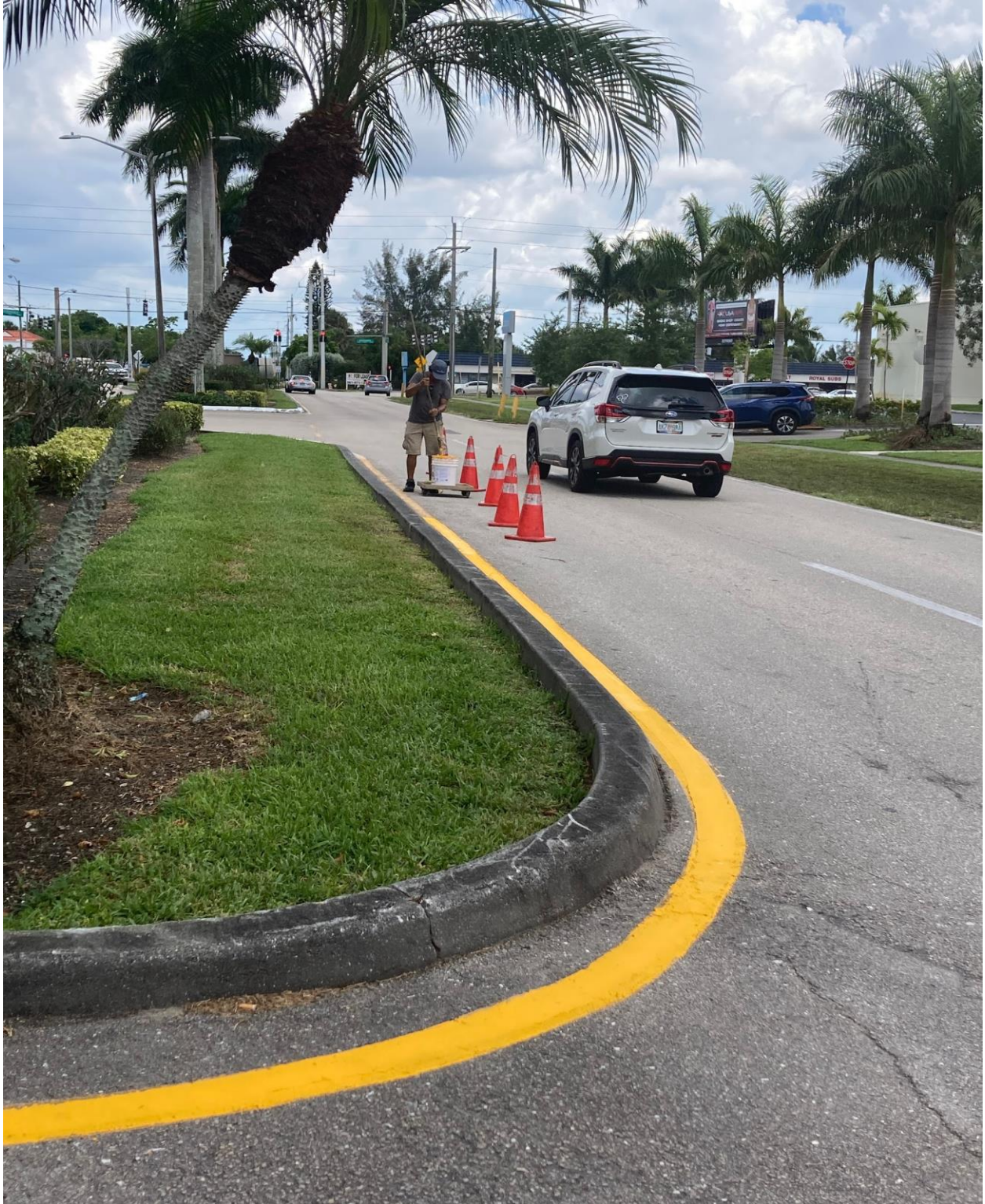
WEST DRIVE- HANDYMAN JOSE CONTINUES WITH ROADWAY PAINTING: CURBS, SPEED BUMPS, STOP BARS. NICE WORK, JOSE.
