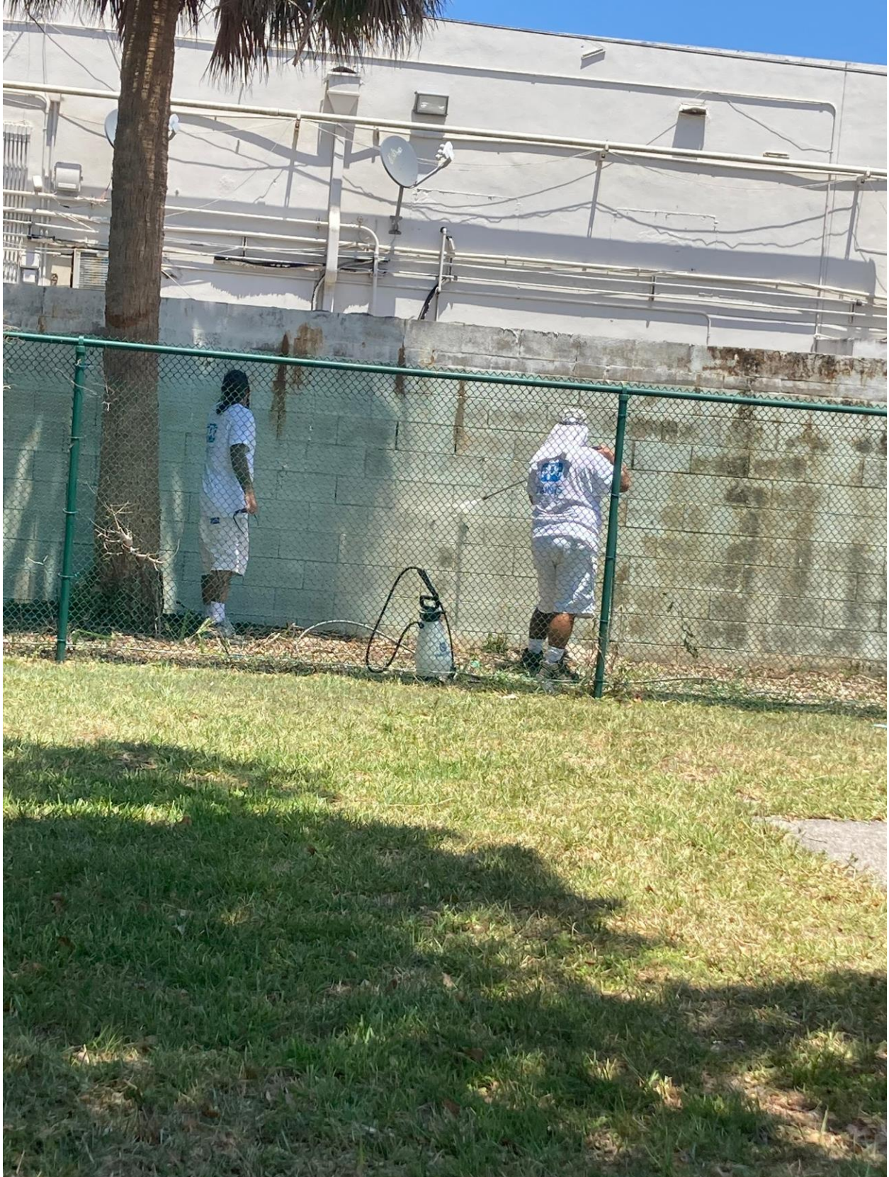
SOUTHAMPTON SECTION- WALL WAS PRESSURE CLEANED ON 6/6.
