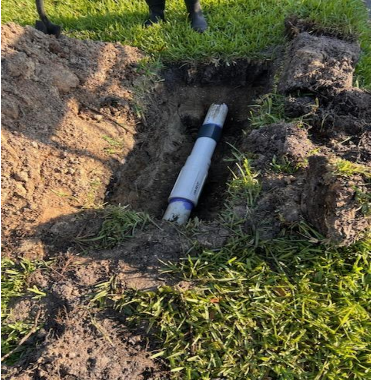
CAMBRIDGE G- FOUR INCH IRRIGATION SUPPLY PIPE REPAIRED BY SEACREST SERVICES.
