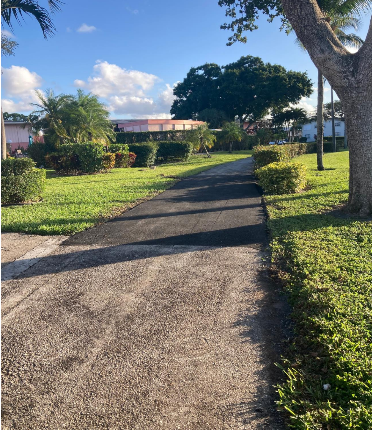
GOLFS EDGE- WALKWAY REPAIR COMPLETE.
