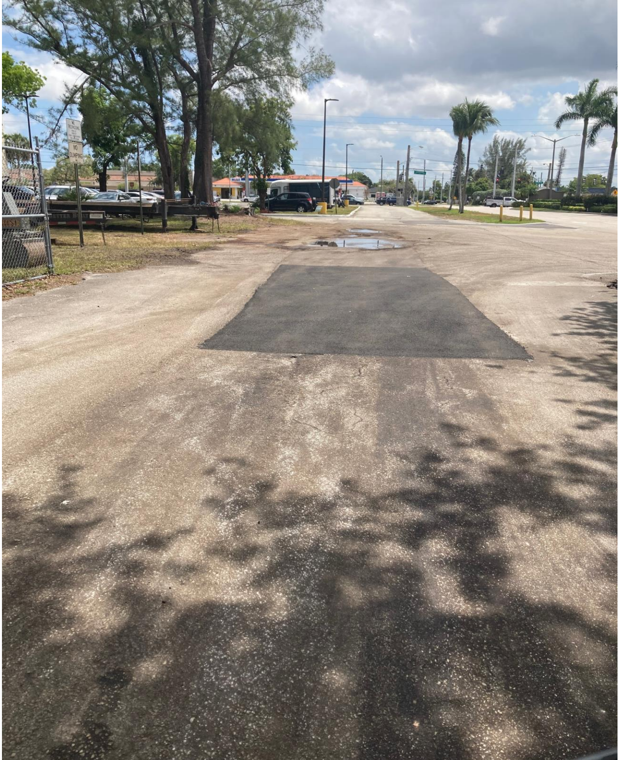
UCO OFFICE- PAVING REPAIR COMPLETE.
