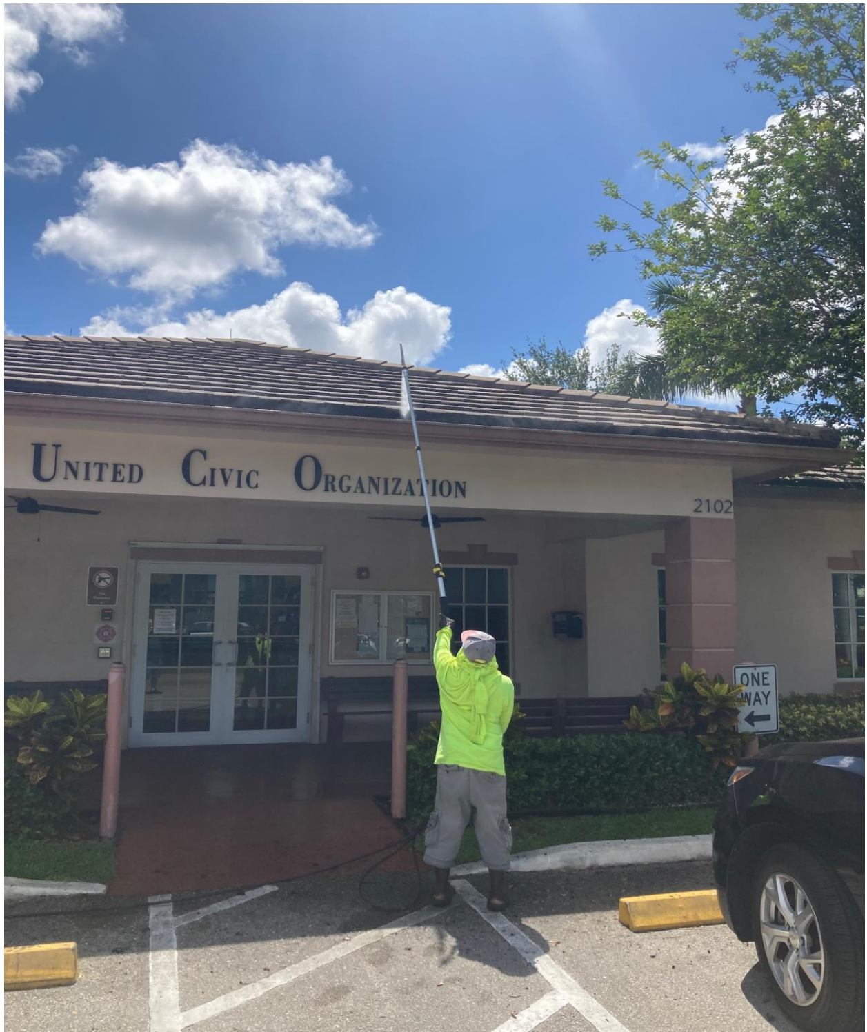
UCO OFFICE- ON 6/6, GLOW CLEANING PLUS CLEANED OUT THE ROOF GUTTERS AT THE UCO OFFICE BUILDING.
