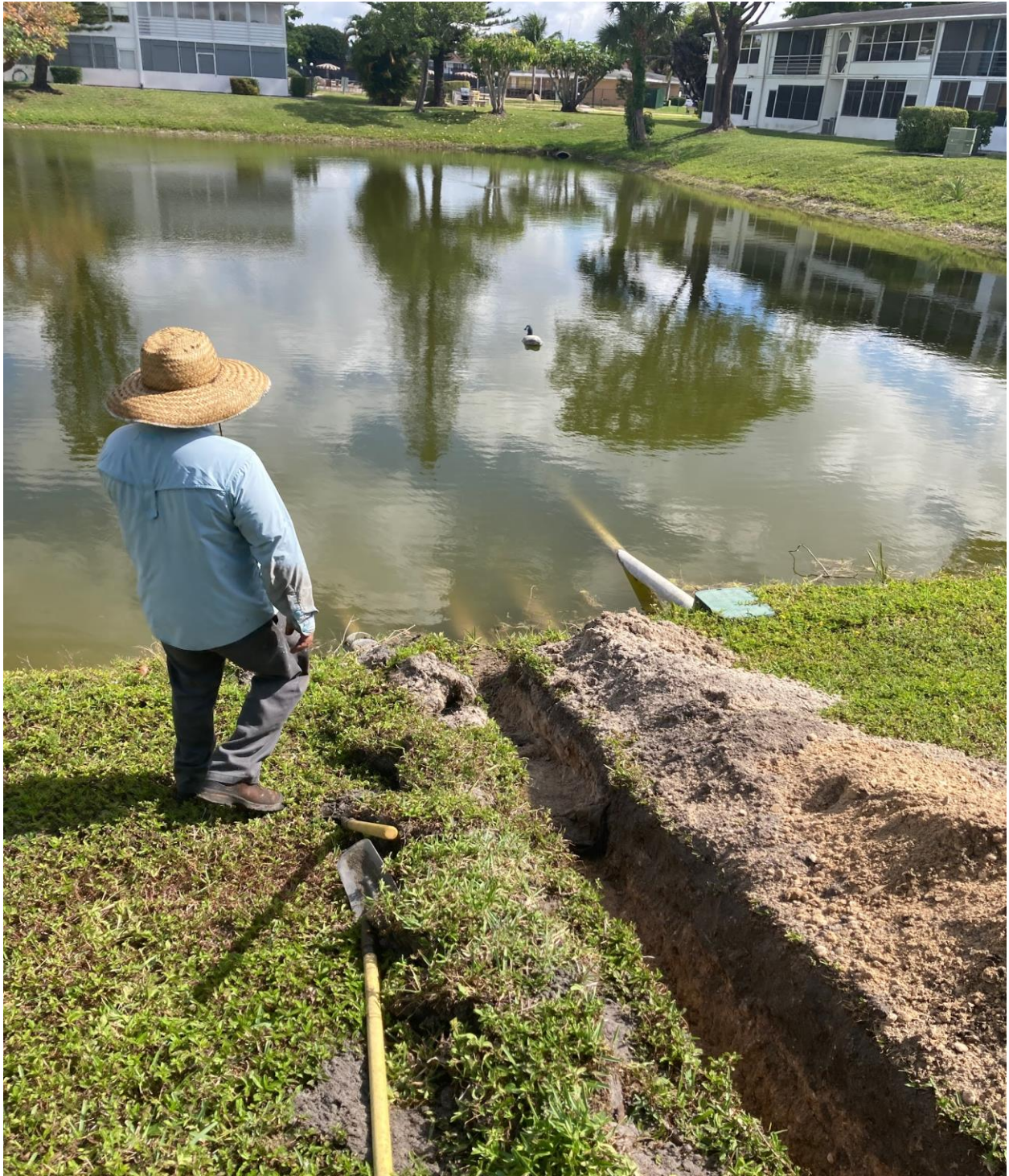
SOMERSET SECTION- ON 6/6, CHABOT IRRIGATION INSTALLED A NEW INTAKE LINE AND CHECK VALVE AT THE SOUTH DRIVE MAIN LOOP IRRIGATION STATION. THIS STATION, ALONG WITH ANOTHER ON NORTH DRIVE, SERVES THE SPRINKLERS ALONG THE MAIN ROADS OF CV.
