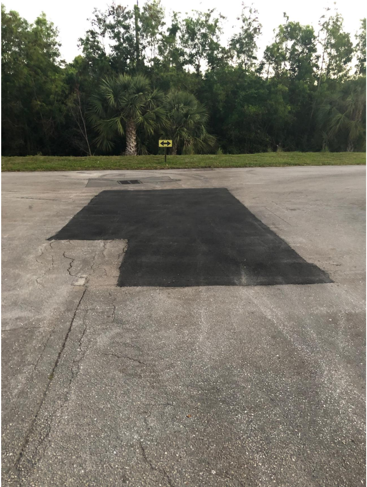
CANTERBURY SECTION- PAVING REPAIR COMPLETE.
