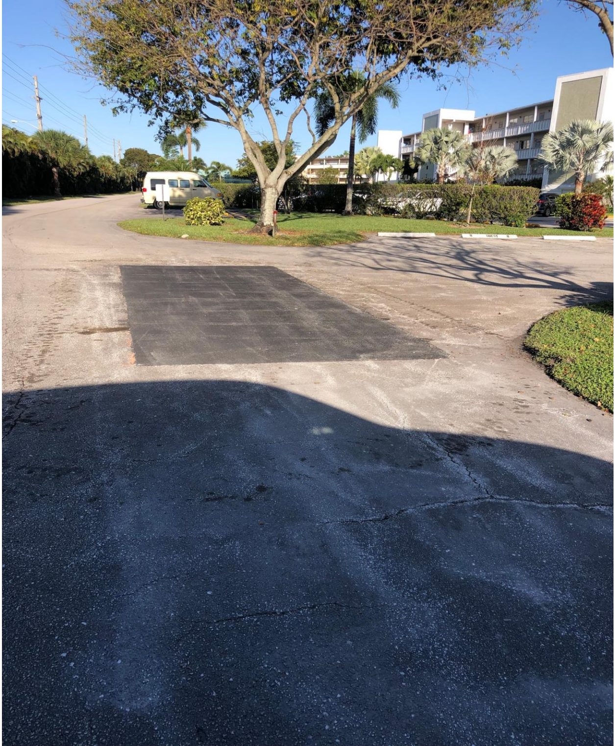
SOUTHAMPTON SECTION- PAVING REPAIR COMPLETE.
