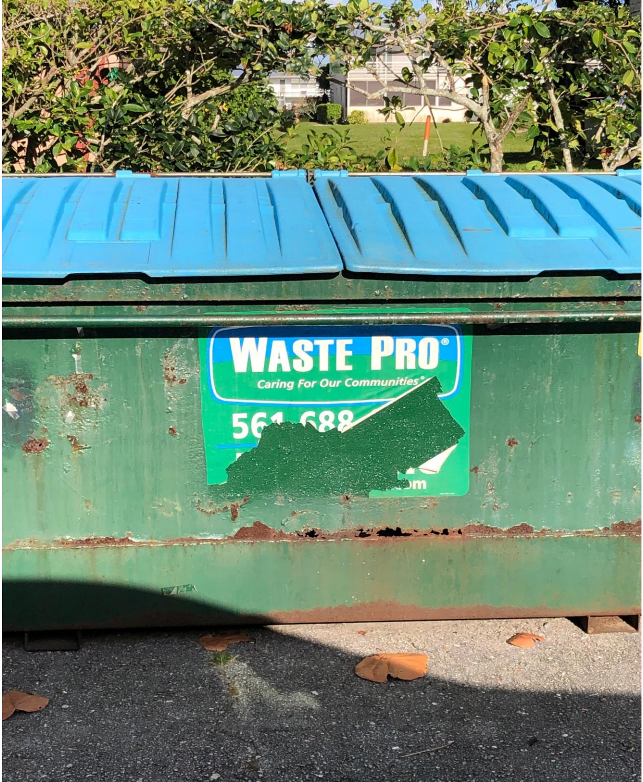
OXFORD 300- HOLEY DUMPSTER, REQUEST FOR REPLACEMENT WAS SENT TO WASTE PRO.
