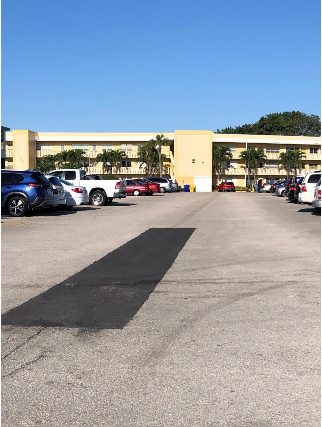
ANDOVER SECTION- PAVING REPAIR COMPLETED.
