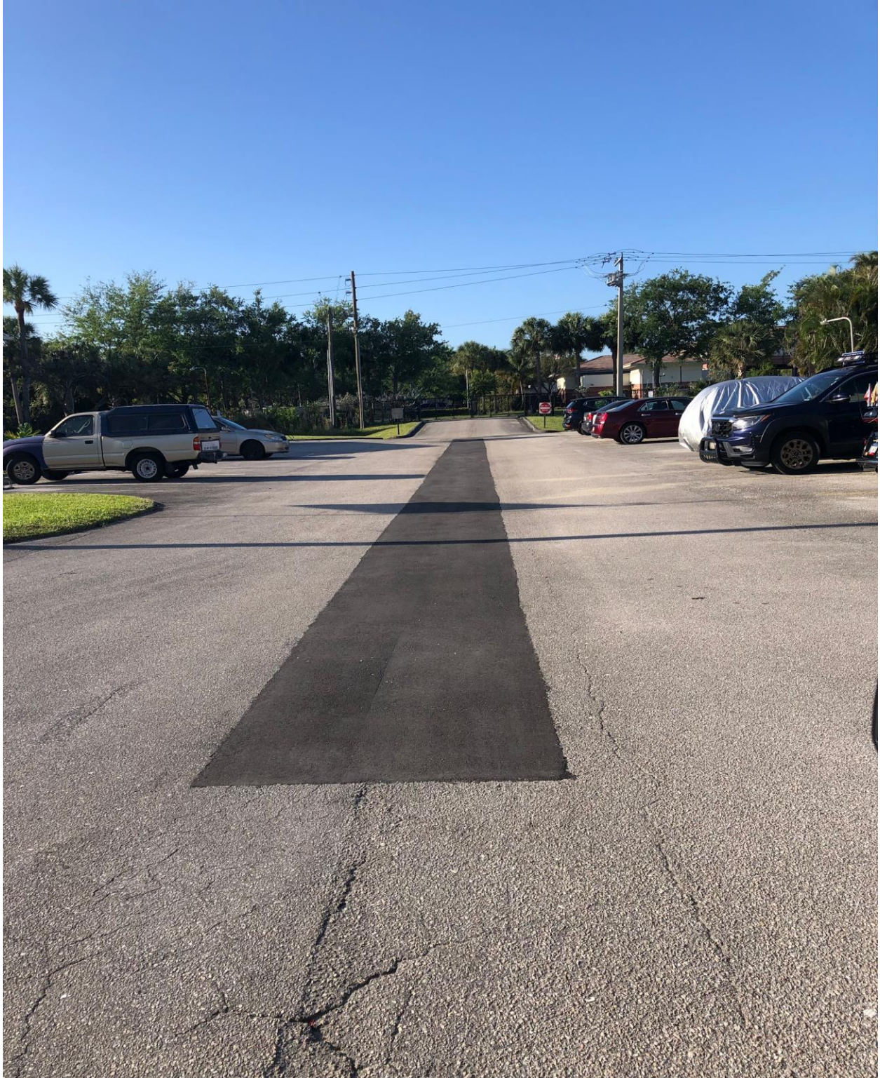
BEDFORD SECTION- PAVING REPAIR COMPLETE.
