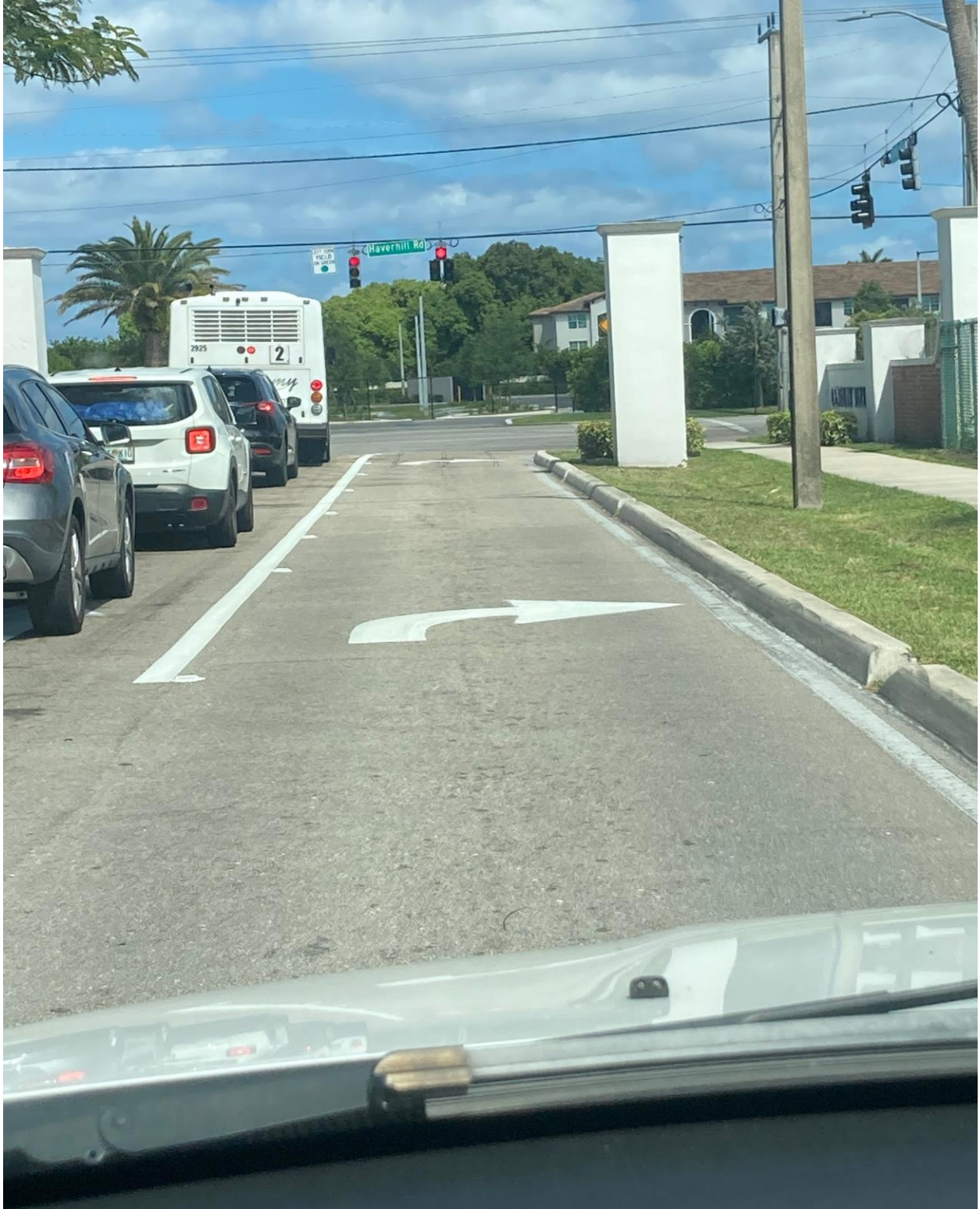
CENTURY BOULEVARD- NEW DIRECTIONAL ARROWS PAINTED BY PBC TRAFFIC DIVISION. RIGHT EXIT LANE IS FOR RIGHT TURNS ONLY.
