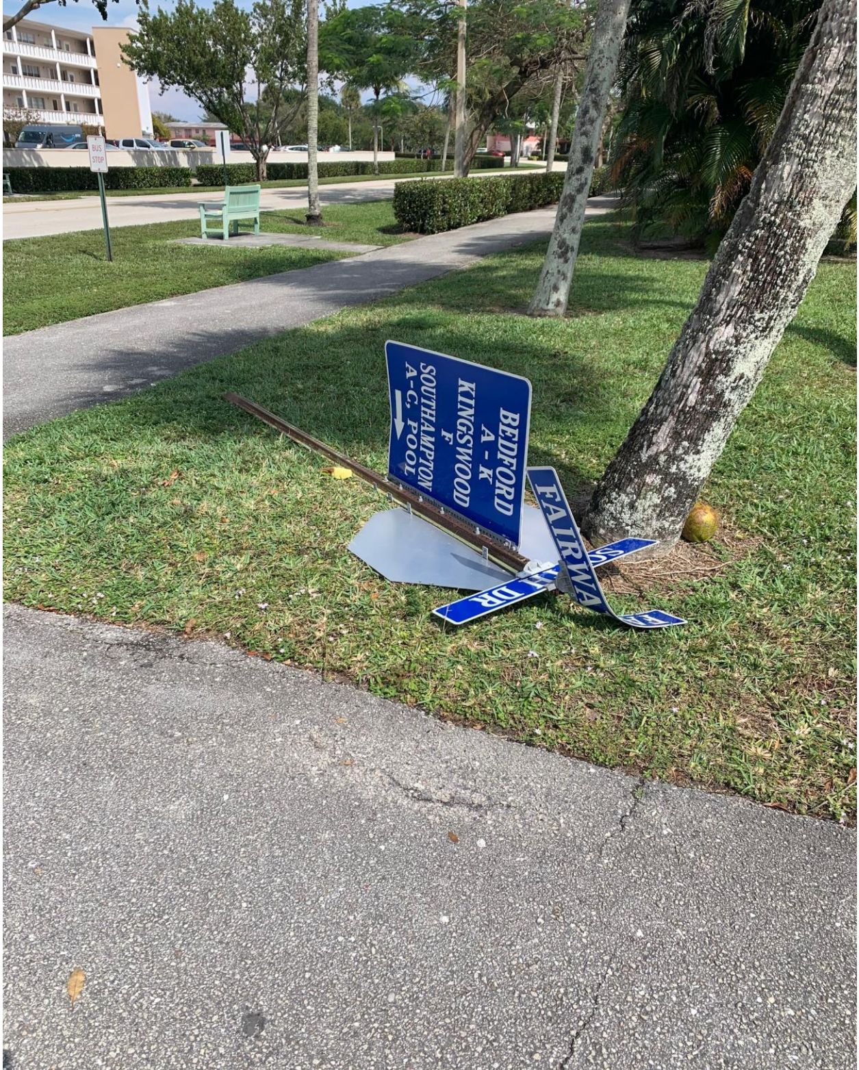
EAST DRIVE- ON 3/7, THIS STREET SIGN POLE WAS KNOCKED DOWN BY A VEHICLE. I NEEDED TO ORDER SOME PARTS, SO THE REPAIR WILL HAPPEN NEXT WEEK.
