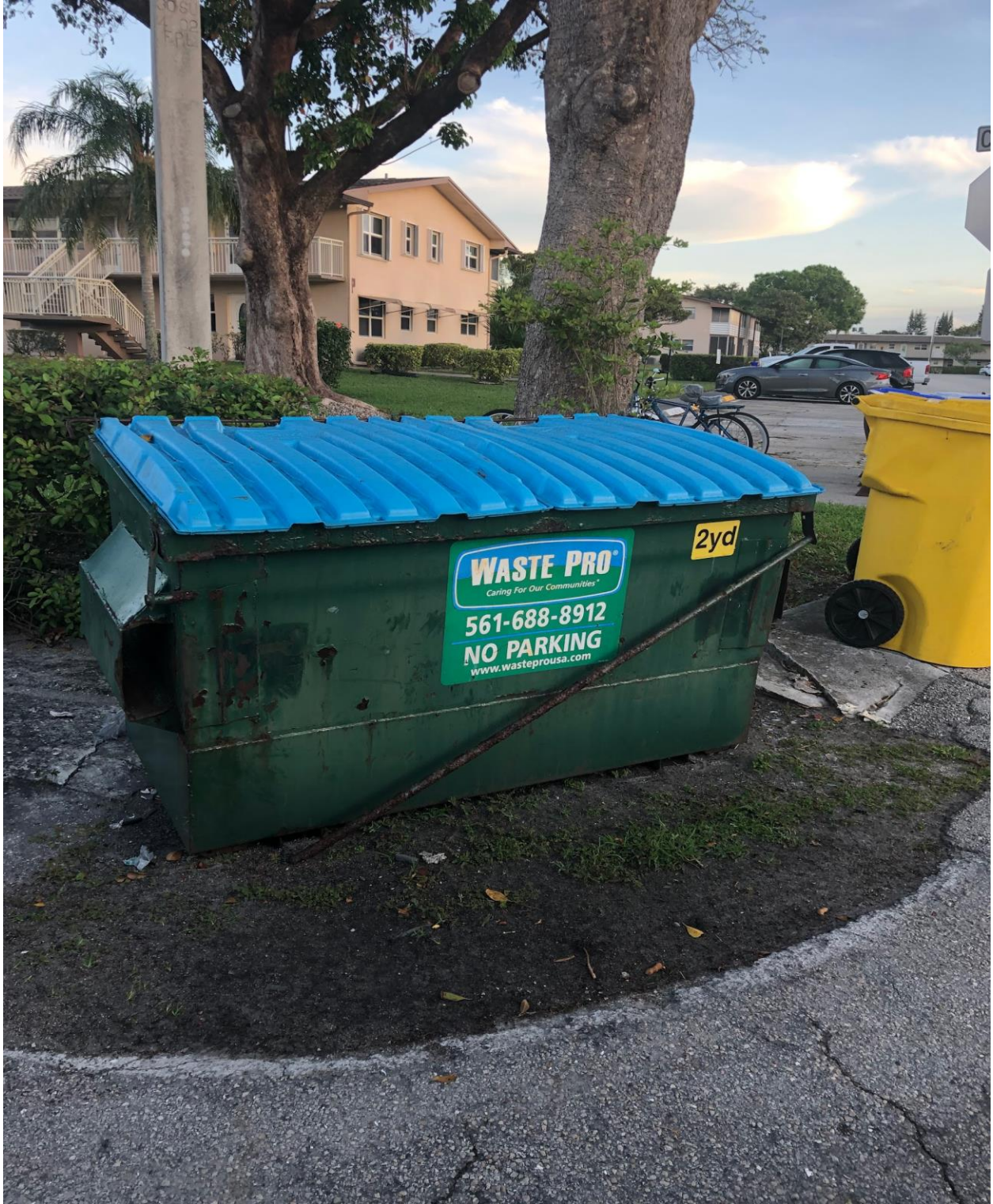
CHATHAM P- BUSTED DUMPSTER. SECOND REQUEST FOR REPLACEMENT SENT TO WASTE PRO.
