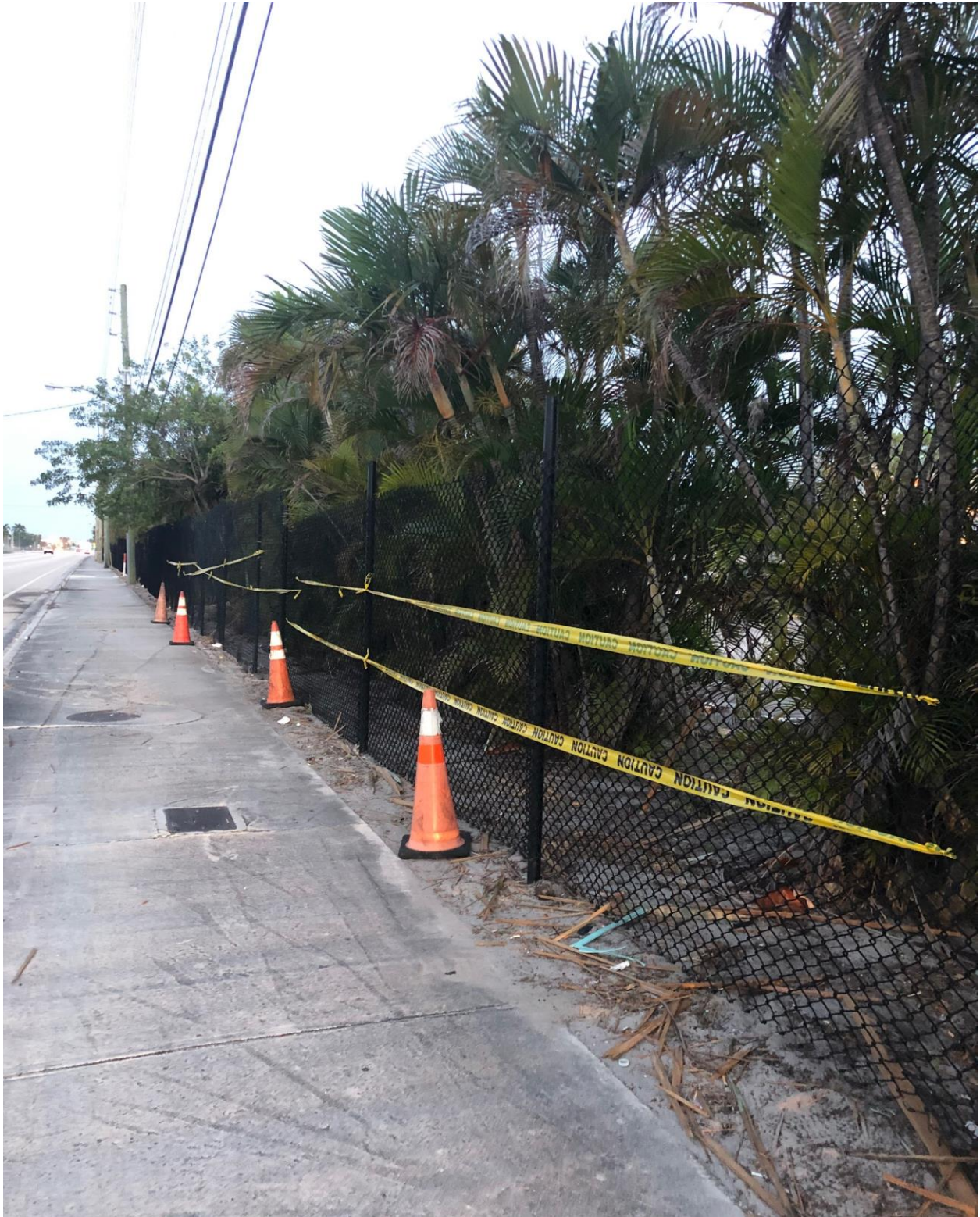
OKEECHOBEE BOULEVARD- TEMPORARY REPAIRS TO PERIMETER FENCE ARE COMPLETE.
