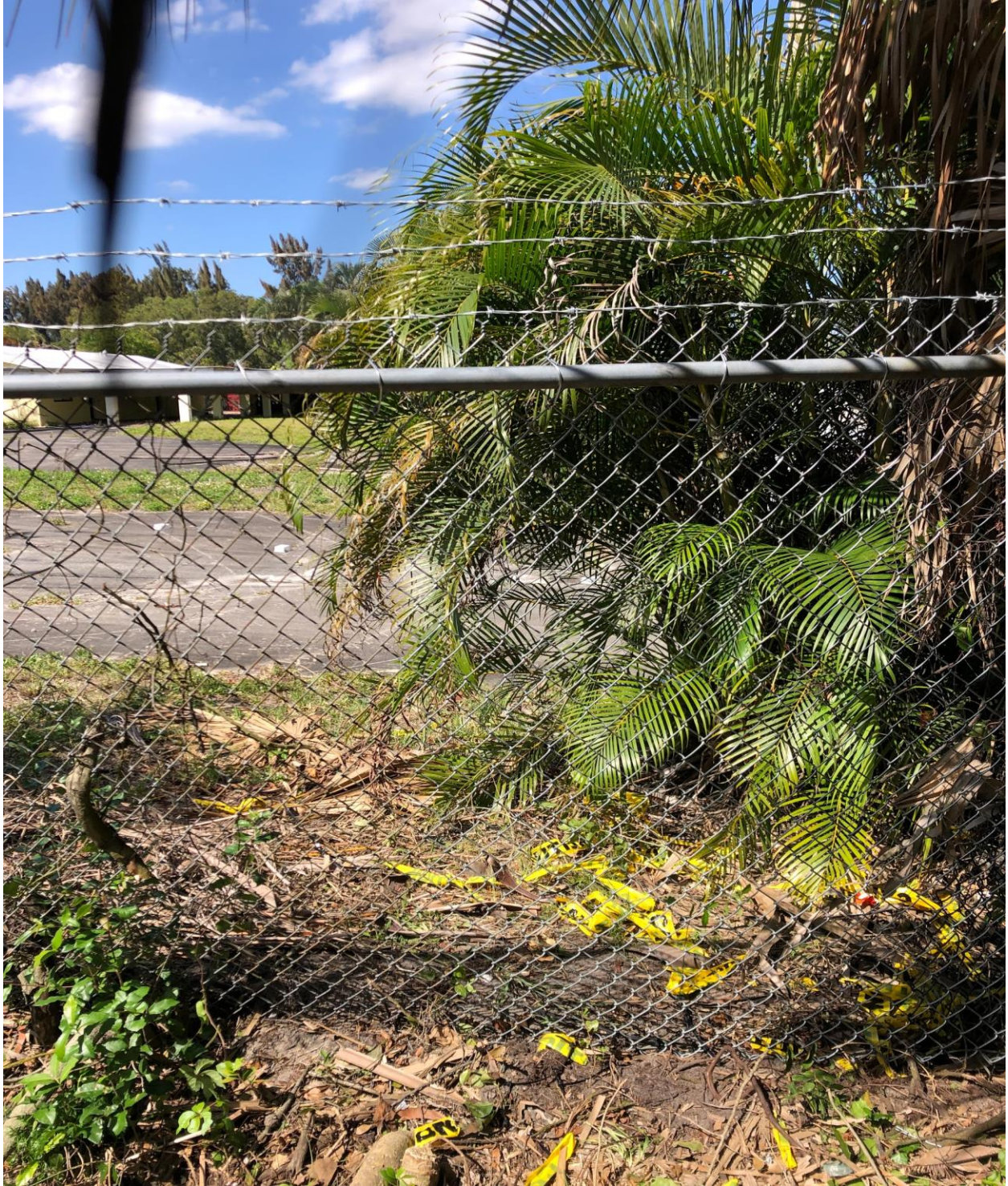
NORWICH SECTION- PERMANENT REPAIRS WERE MADE TO THIS FENCE BY BUDGET FENCE AND GATE ON 3/20.
