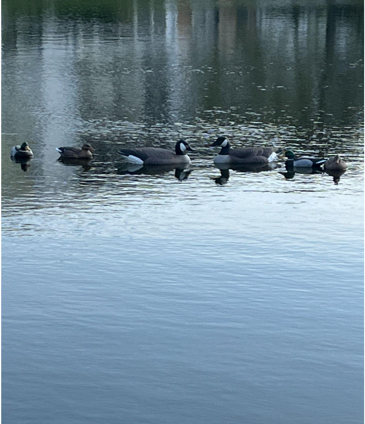
LAKE WELLINGTON- THESE PLASTIC DUCKS AND GEESE WERE INSTALLED BY CHABOT IRRIGATION LAST WEEK. THEIR JOB IS TO HOLD A BELOW-WATER IRRIGATION PUMP INTAKE PIPE UP AND OUT OF THE MUD.
