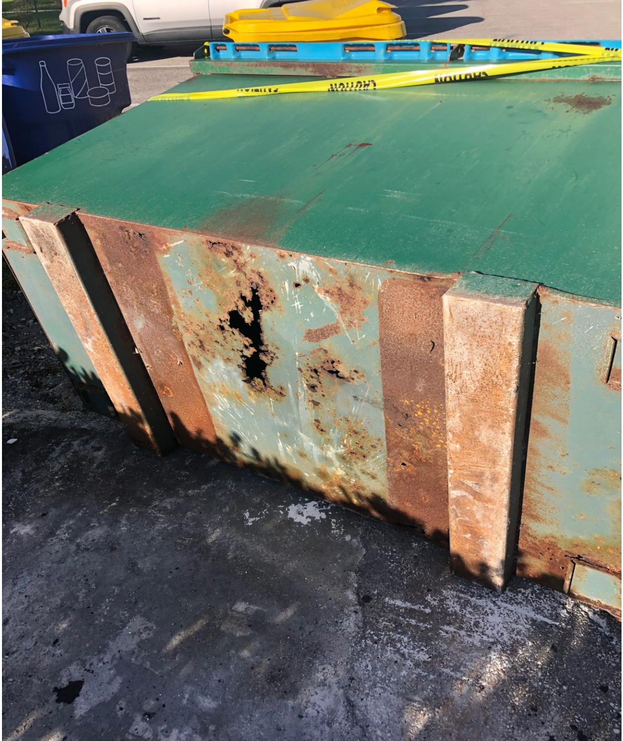
BEDFORD G- ROTTED OUT DUMPSTER. REQUEST FOR REPLACEMENT WAS SENT TO WASTE PRO.
