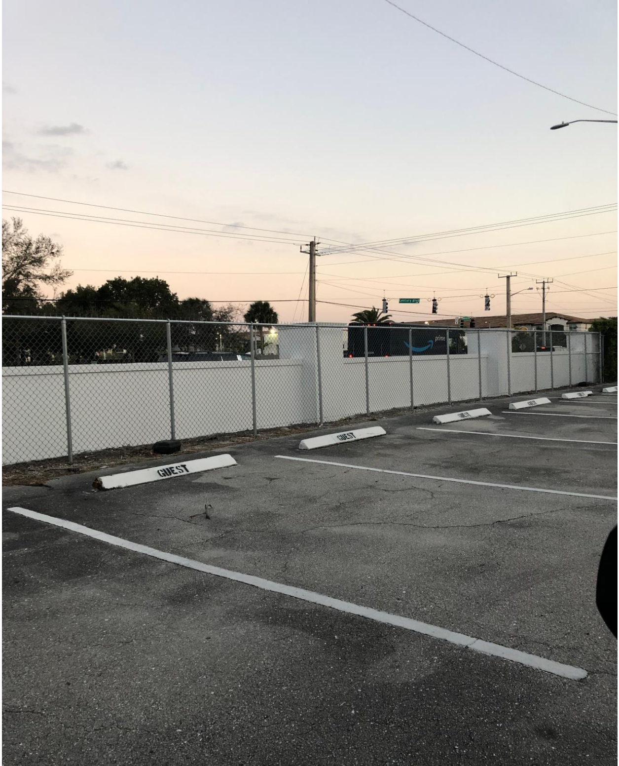
EASTHAMPTON SECTION- MASONRY WALL PAINTING COMPLETE, FENCES HAVE BEEN REINSTALLED.
