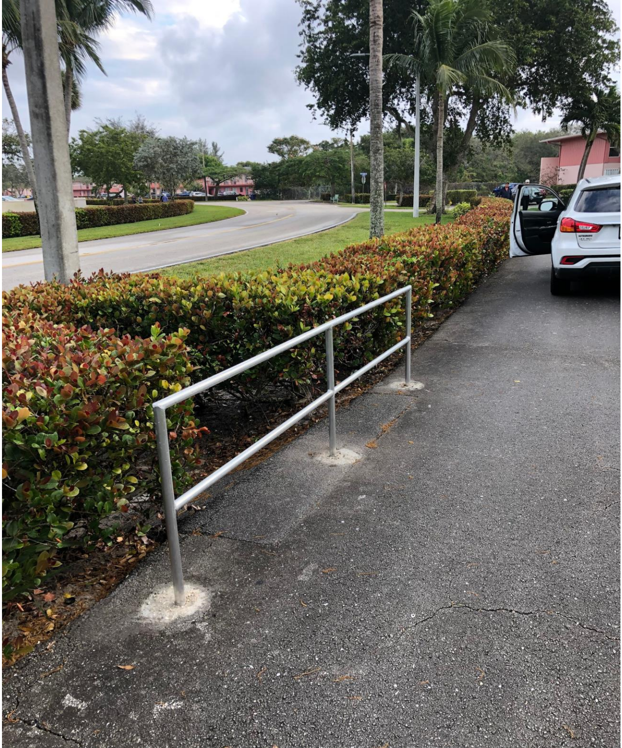
EAST DRIVE- RAILING REPAIR COMPLETE.
