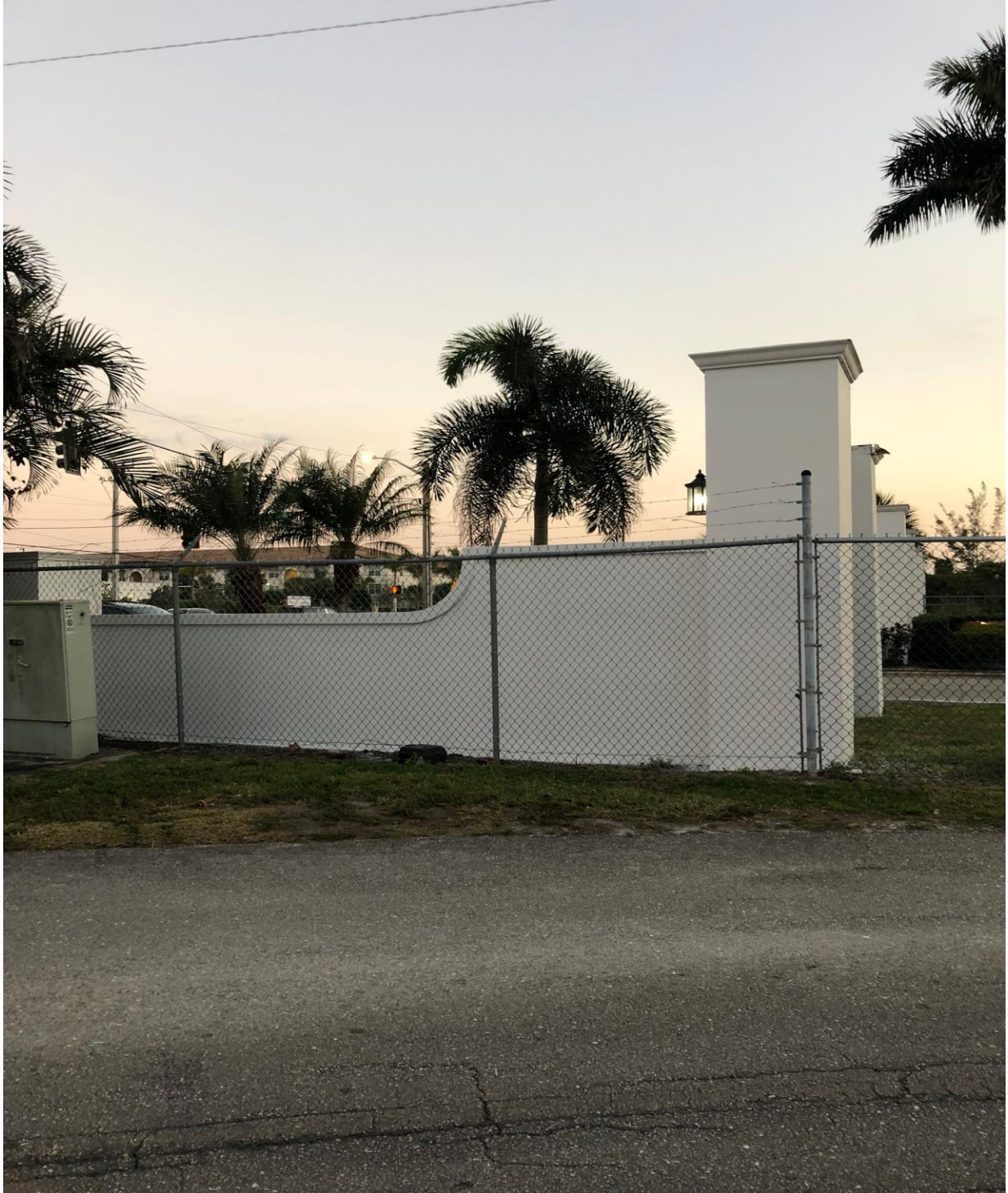
EASTHAMPTON SECTION- MASONRY WALL PAINTING COMPLETE, FENCE HAS BEEN REINSTALLED.
