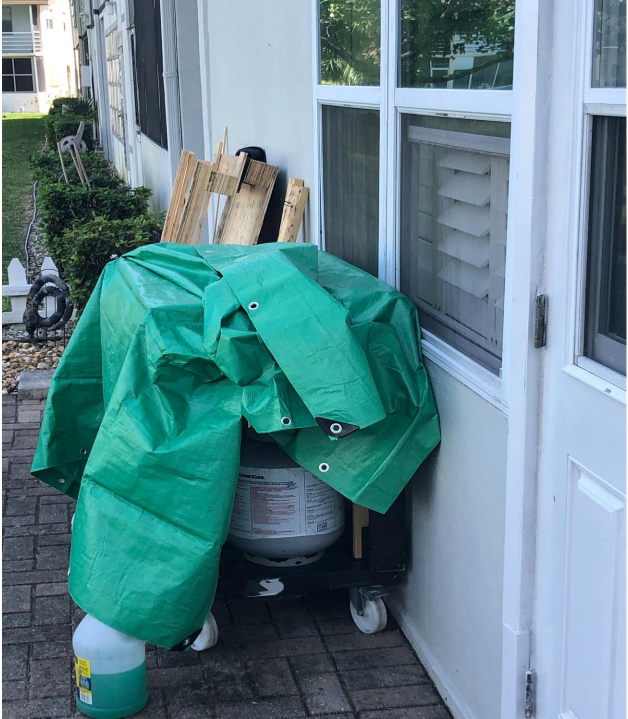
NORTHAMPTON K- PROPANE TANK UP AGAINST THE BUILDING. REPORTED TO UCO BY A NORTHAMPTON K UNIT OWNER. THIS IS DANGEROUS. A REPORT WAS SENT TO PBC CODE ENFORCEMENT, COMPLAINT # C-2024-02130019. THE ASSOCIATION'S PROPERTY MANAGER WAS NOTIFIED.
