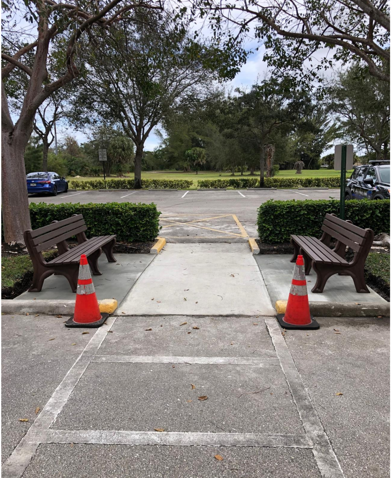
UCO OFFICE- NOW THE SITTING AREA IS LEVEL.
