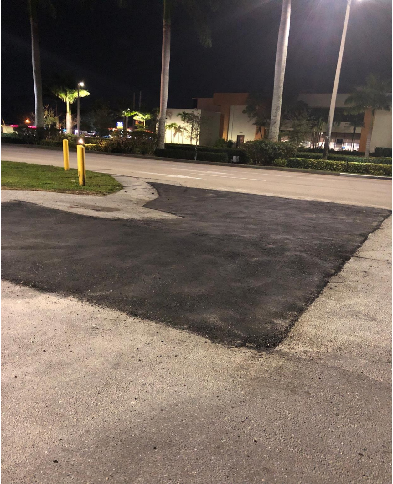
WEST DRIVE- PAVING REPAIRS AT WELLS FARGO BUILDING COMPLETED ON 1/7.
