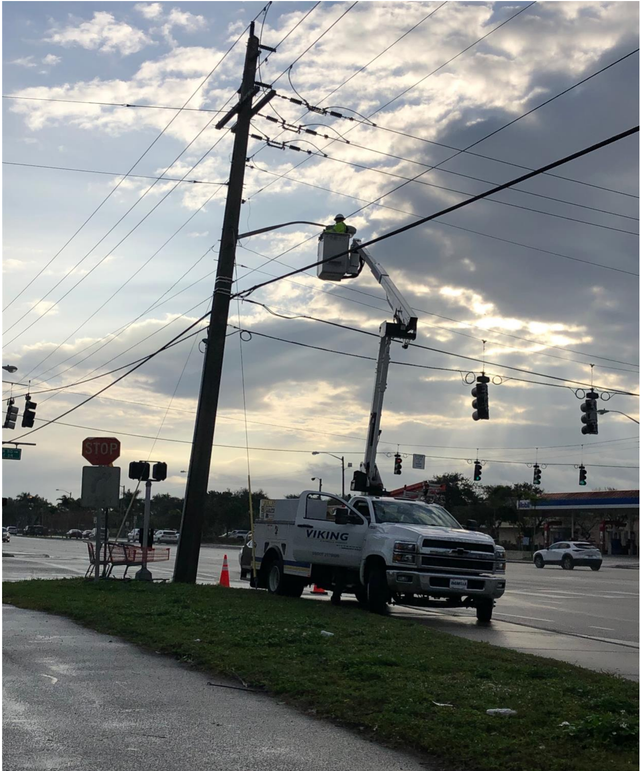
OKEECHOBEE BOULEVARD- THIS STREET LIGHT WAS REPAIRED ON 1/12.
