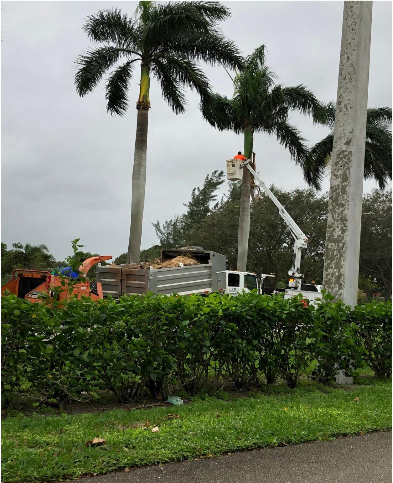
CENTURY BOULEVARD- ON 12/16, D.R. LAWN SERVICE COMPLETED TRIMMING OF PALMS ALONG THE MAIN ROADS OF CV. JUST IN TIME FOR THE STORM.
